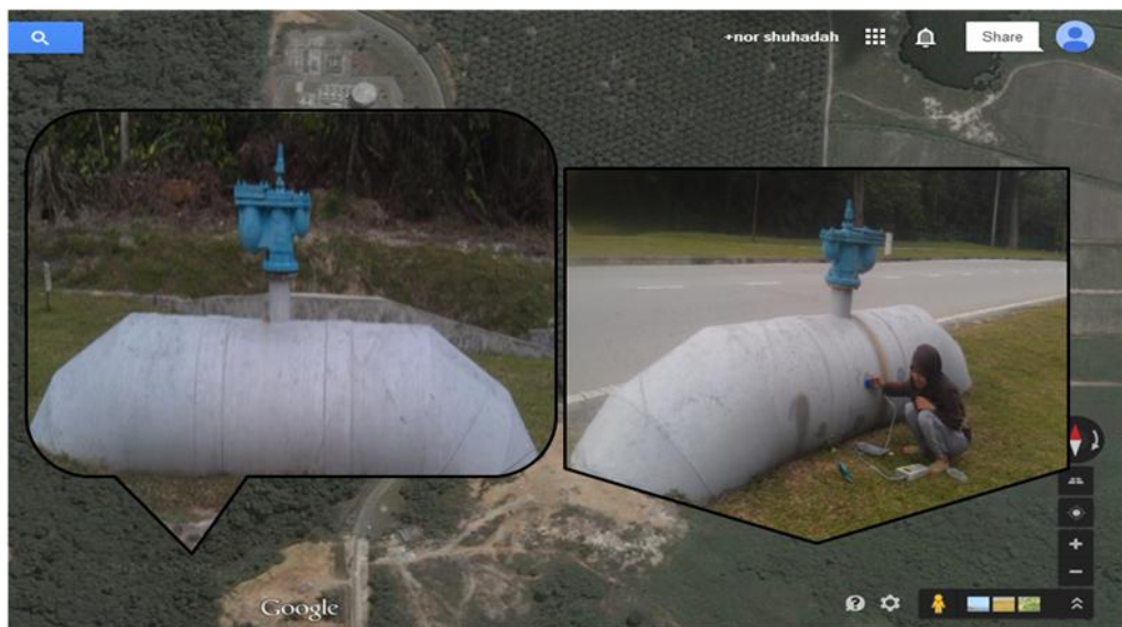
Figure 10: Pipeline near to GDC
