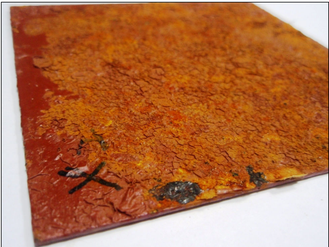
Specimen E2-U – Blisters and lost of adhesion failures
