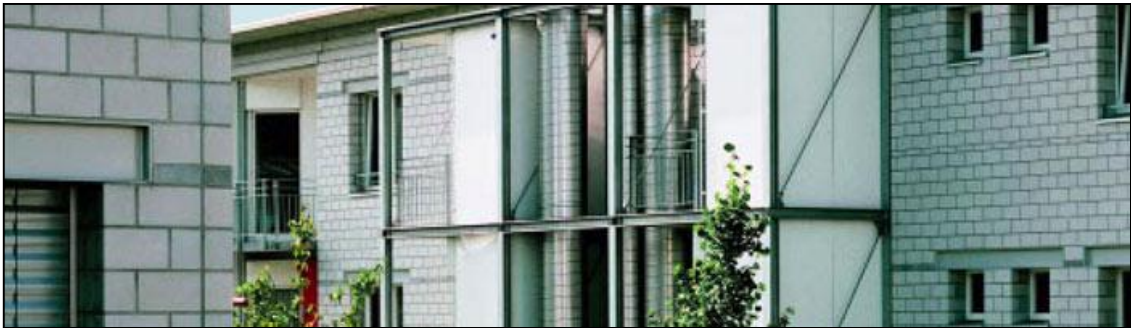
Figure 2: the application of Sand – Lime Brick
