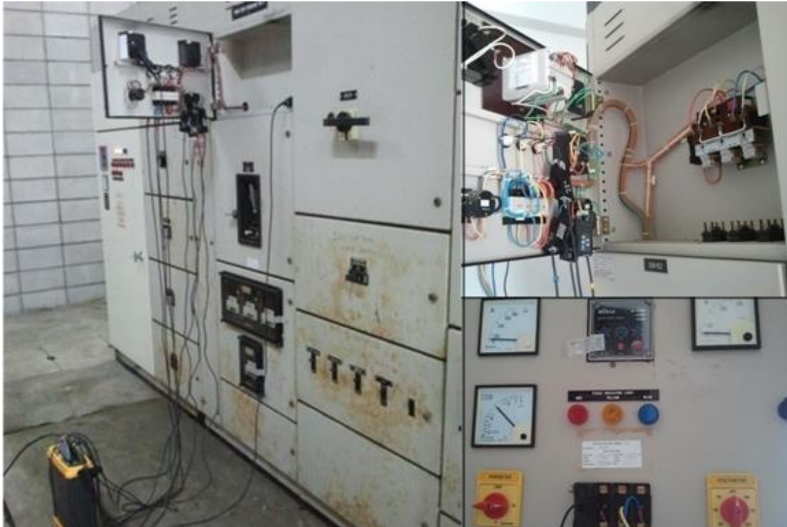
Figure 3.5 Fluke 1750 power analyser logging data at SSB V31
