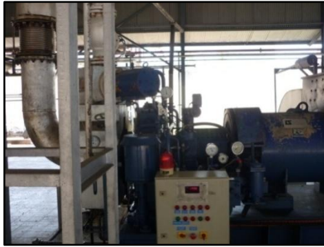
Figure 2.1: Turbine, facing north
