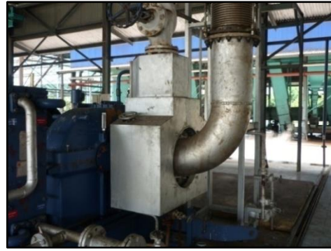
Figure 2.2: Turbine, facing south
