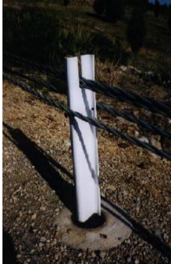
Figure 15.0: The exposed post area
