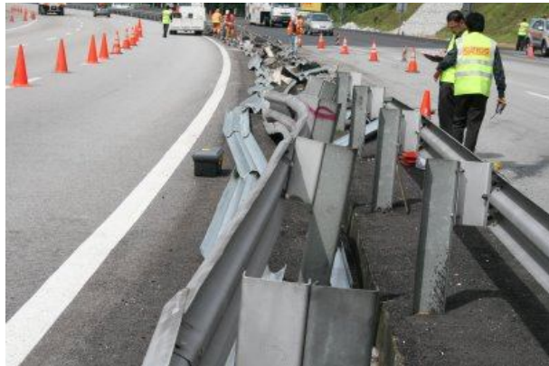
Figure 1: Broken guardrail from the Rawang express bus accident ( http://transitmy.org/2009/12/26/sani-express-tragedy-have-we-learned-anything/ )
