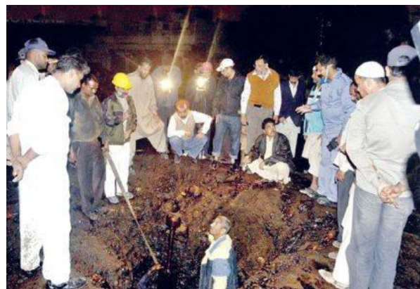
Figure 2.22: Pipeline of Parco Burst in Korangi Karachi.
