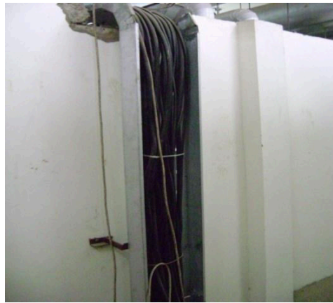
Figure 2.32: Uncovered Electrical Cable Trench in Power Generation Room.
