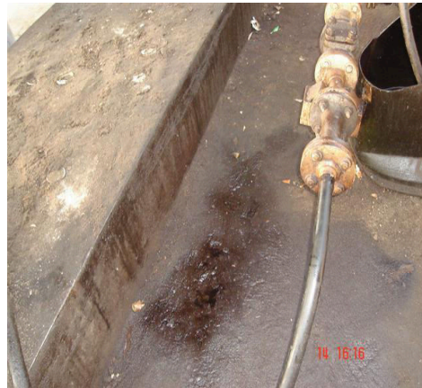
Figure 2.36: Spillage at Additive Dosing Point
