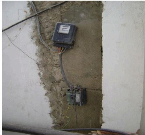
Figure 2.30: Unsafe Electrical Connections in Power Generation Room.
