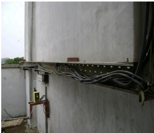
Figure 2.33: Uncovered Electrical Trench.
