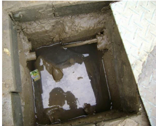
Figure 2.18: Cable Trench was found Filled with Water.
