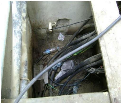
Figure 2.31: Electric Cables Trench was found Uncovered. Cables found Irregular.
