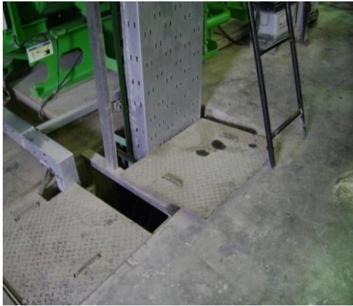
Figure 2.29: Cable Trays were not Properly Covered.
