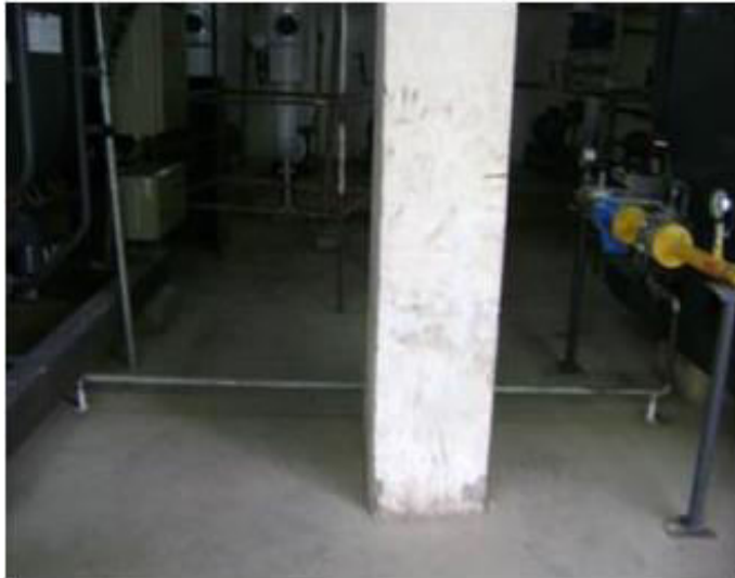
Figure 2.23: Diesel Dozing Pipe has become a Trip Hazard
