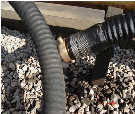
Figure 2.35: Use of Non-standardized Couplings at PFS.
