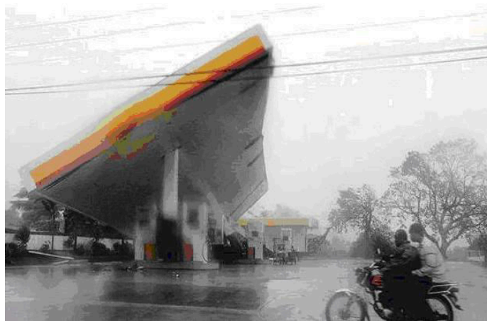
Figure 2.7: The Roof of a Petrol Station gets Damaged by Typhoon Megi in Isabela Province, Northern Philippines. (19 th October, 2010)
