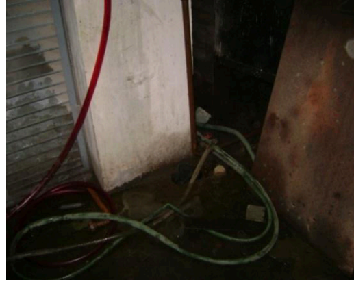
Figure 2.16: Spillage Marks in Power Generation Room.
