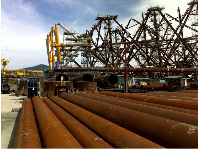
Figure 3.2: Fabrication yard in Malaysia
