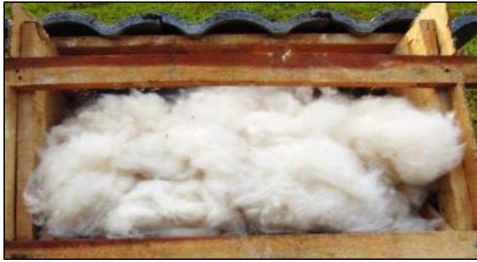
Figure 3.9: Installation of insulation material in roof structure
