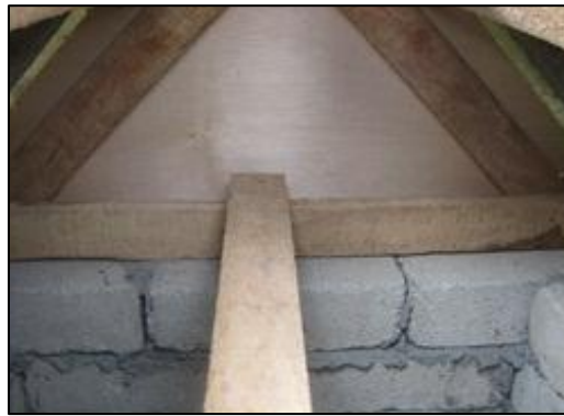
Figure 3.7: Placement of roof structure on top of brick wall (interior side view)
