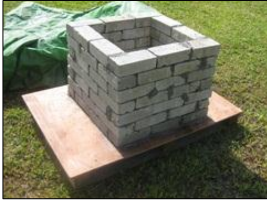
Figure 3.6: 125-mm thick concrete brick wall with no finishing
