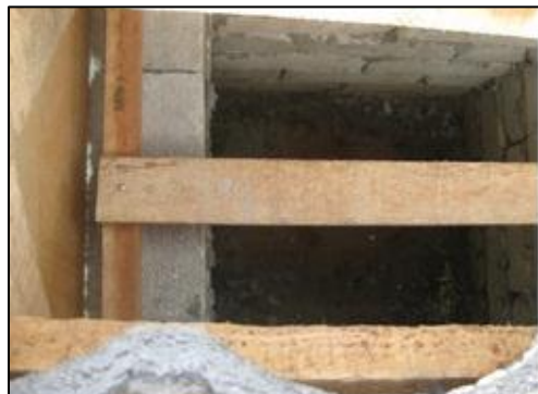
Figure 3.8: Placement of roof structure on top of brick wall (interior top view)
