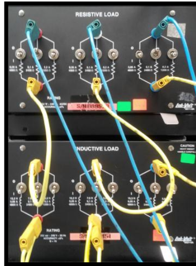
Figure 5: Load settings on EMS workstation
