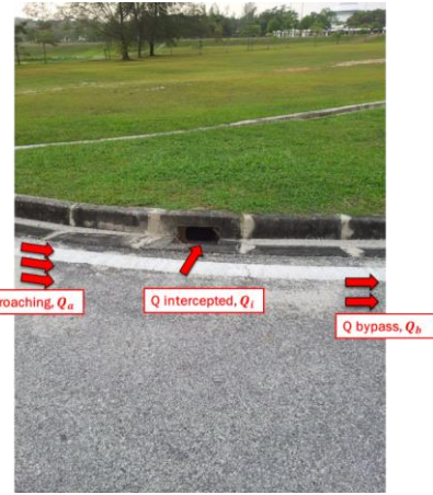
Figure 9: Flow of surface runoff
