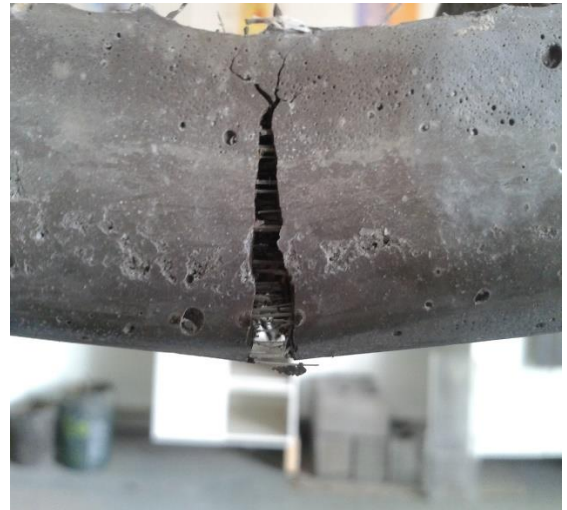
Figure 4.13. Large Crack on specific
