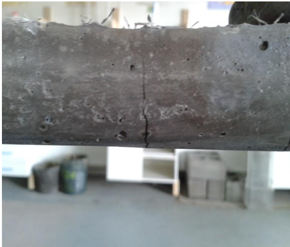
Figure 4.12 Small crack on specific time time
