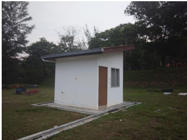
Figure 3.2 – Single room test house inside UTP Campus, before the installation of thermoelectric (TE) air-duct.
