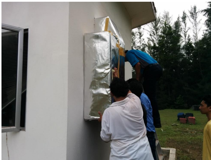
Figure 3.12: Installation of TE air-duct at single test room house
