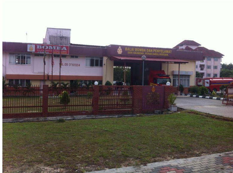
Figure 4.1: Sri Iskandar Fire Station
