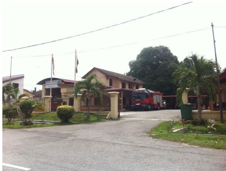
Figure 4.2: Batu Gajah Fire Station
