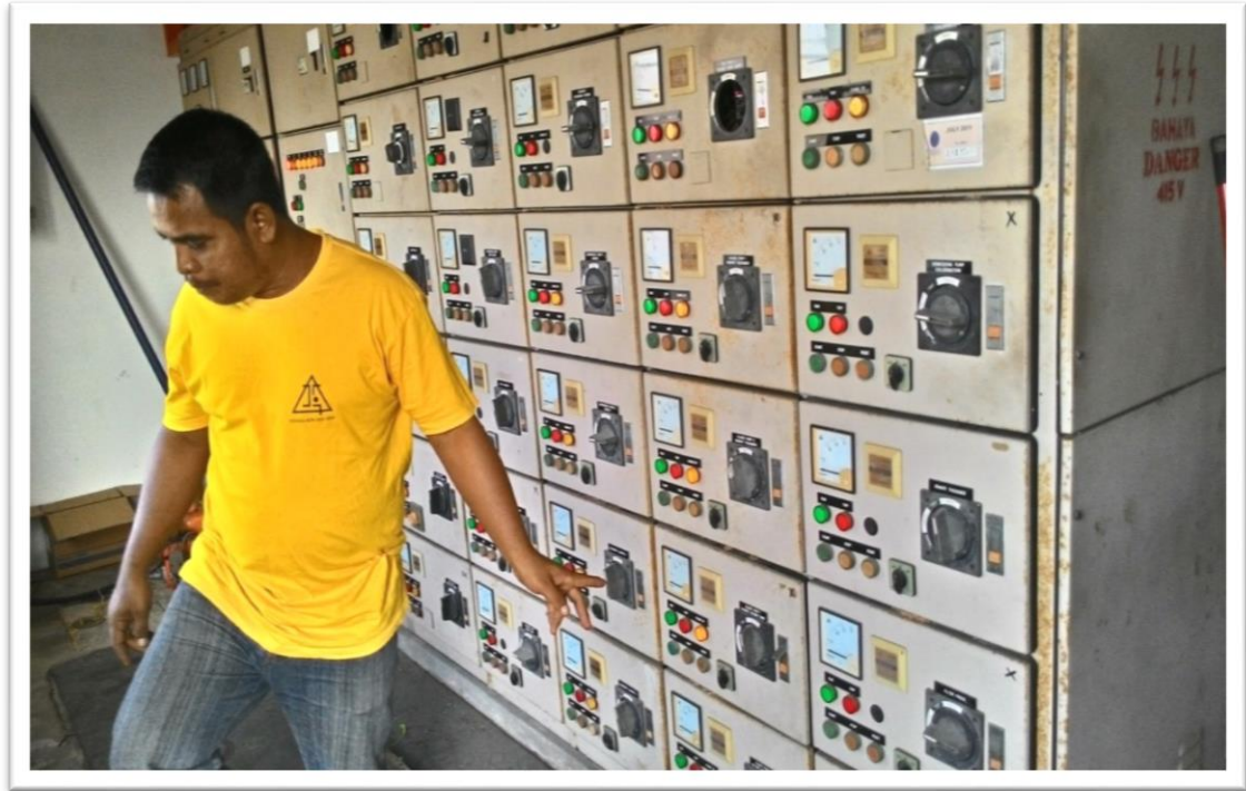
Figure 47 : Operator do some checking on the suizes
