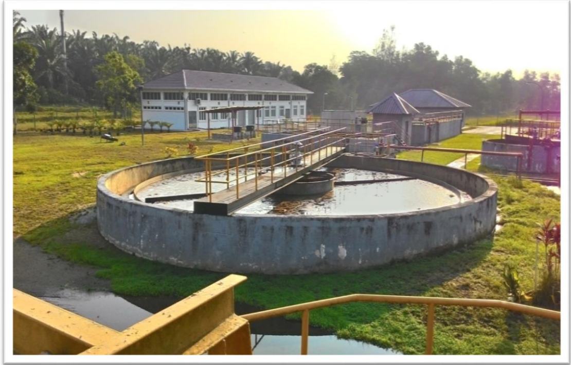
Figure 45: Clarifier 1 (Main UTP STP)
