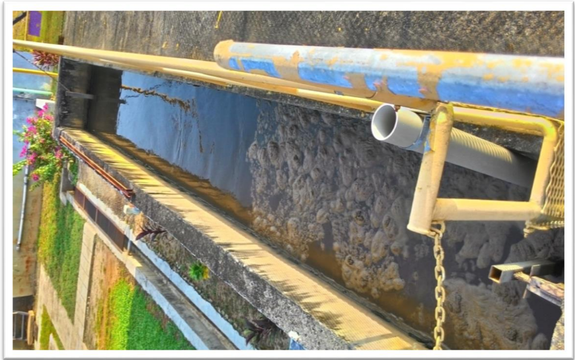
Figure 43 : Anoxic tank (Main UTP STP)
