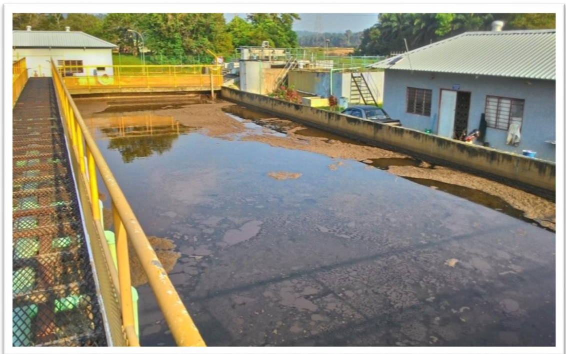
Figure 43 : Anoxic tank (Main UTP STP)
