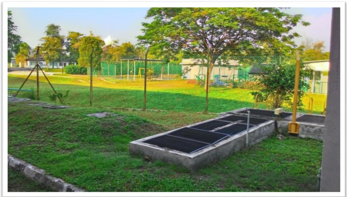
Figure 40 : STP at Block B
