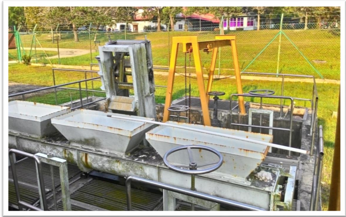
Figure 41: Bar Screen (Main UTP STP)
