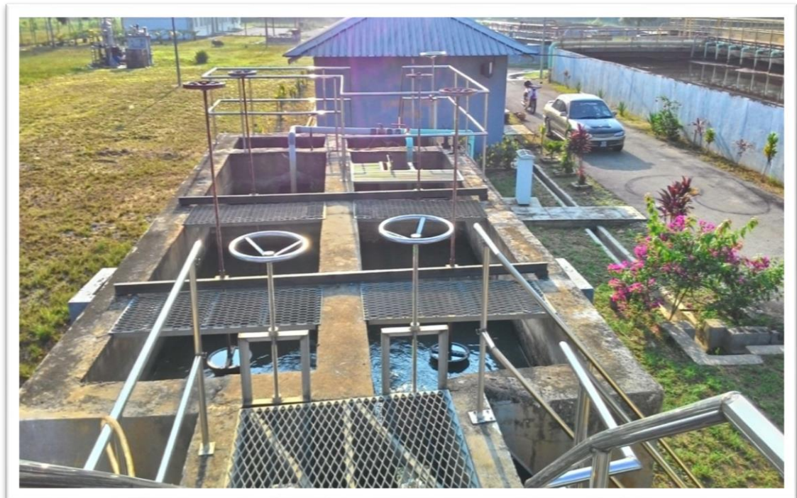
Figure 42 : Grease Chamber (Main UTP STP)
