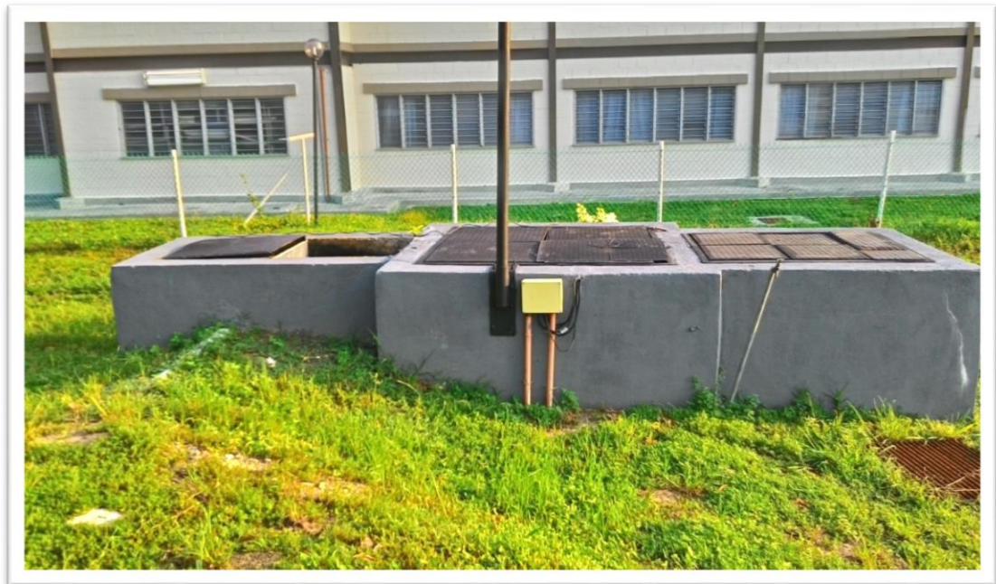
Figure 4 : Screen Chamber of Duyung's STP
