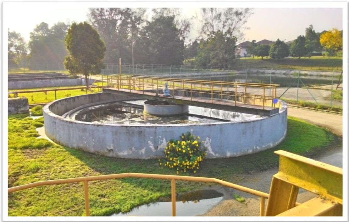
Figure 46 : Clarifier 2 (Main UTP STP)
