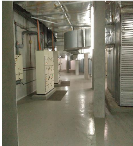
Figure 4.1: Cooling System Unit (Basement)
