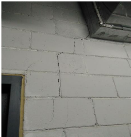
Figure 4.3: Visible Crack (Basement)
