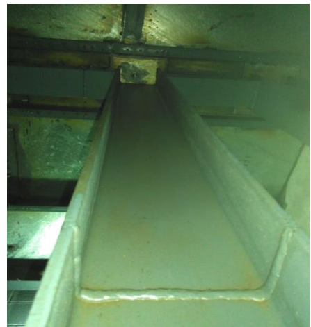
Figure 4.4: Smooth Steel Welding (Basement)
