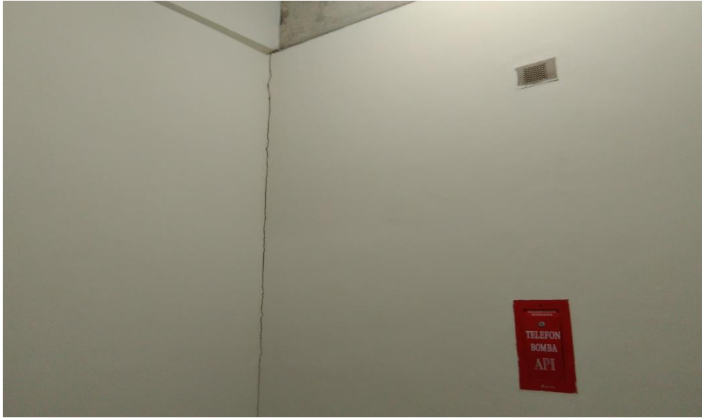
Figure 4.5: Joint Crack visible on one of the room inside Chancellor Hall. (Ground level)
