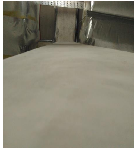
Figure 4.2: Smooth Column (Basement)
