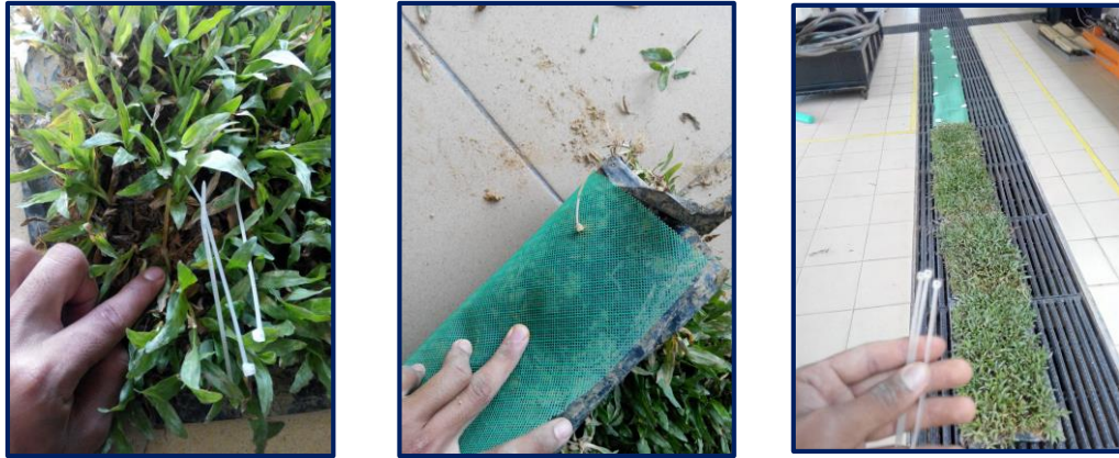
Figure 3.3: Tying vegetation strip onto 10m plastic mesh
