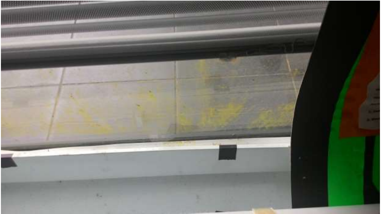
Diagram 31: Mould contamination found on windows at the building exterior ( captured inside the office room )
