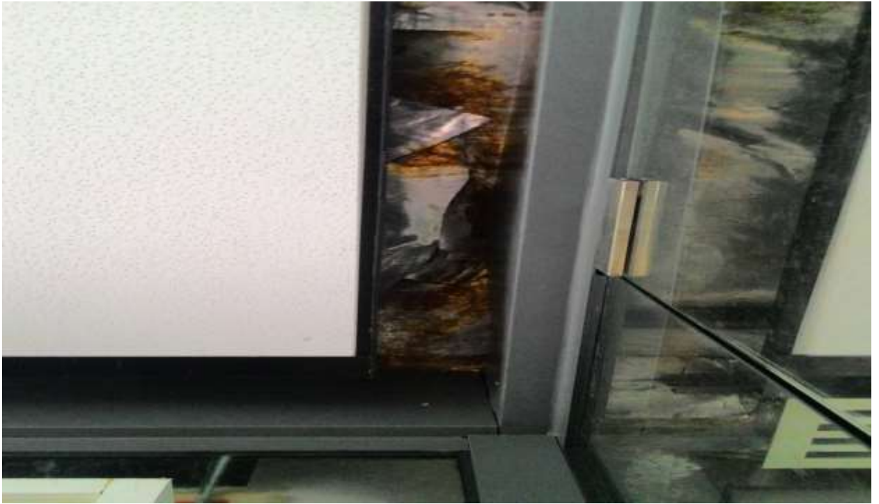
Diagram 25: Discoloration of fibrous insulation
