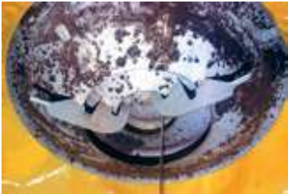
Figure 12: Mould growth on air diffuser in ceiling (Owners, 2006)
