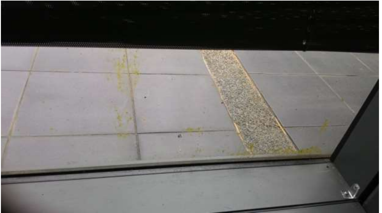
Diagram 33: Mould contamination found on windows at the building exterior ( captured inside the office room )
