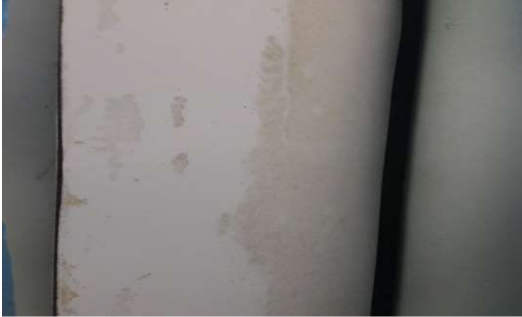
Diagram 19: Mould found at the exterior of cupboards
