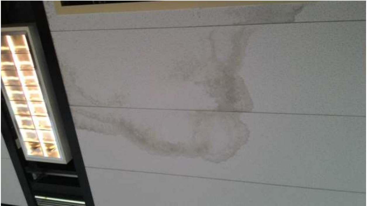
Diagram 9: Water seepage marks found at the ceiling
