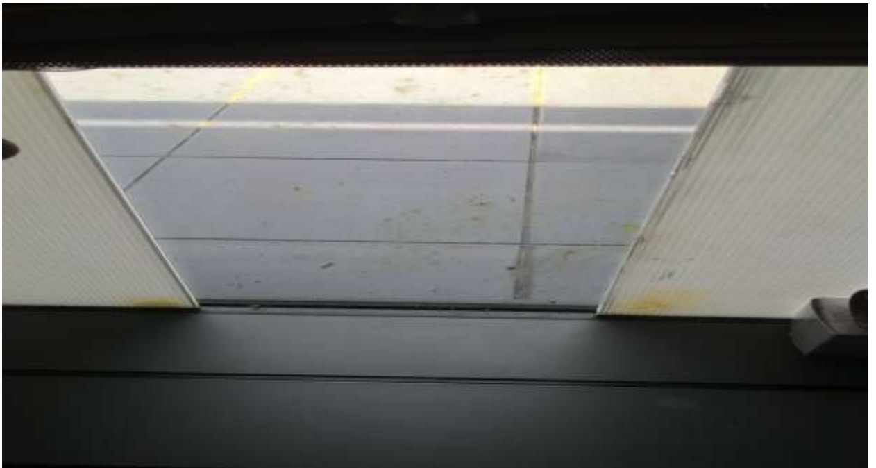
Diagram 32: Mould contamination found on windows at the building exterior ( captured inside the office room )
