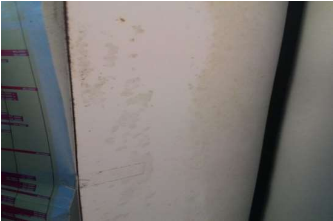
Diagram 20: Mould found at the exterior of cupboards
