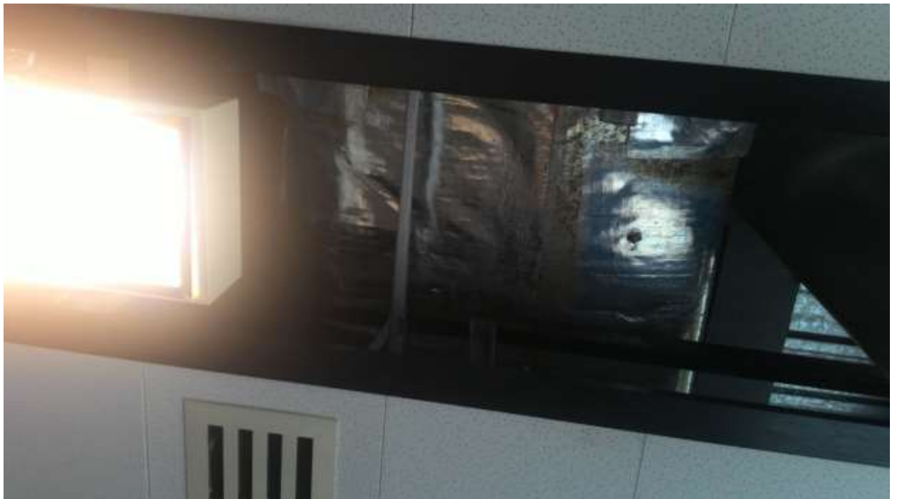
Diagram 24: Discoloration of fibrous insulation
