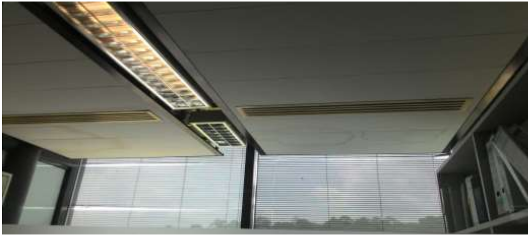
Diagram 3: Plasterboard material used for ceiling and optiwhite type of glass window is used both inside and outside the lecturers room
