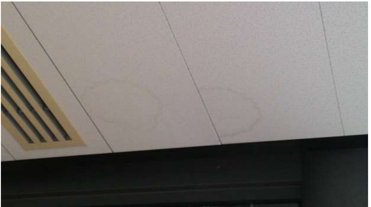
Diagram 10: Water seepage marks found at the ceiling
