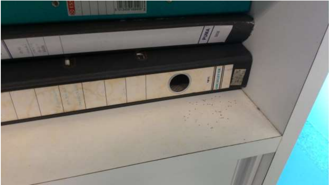
Diagram 23: Mould found at the interior of cupboards
