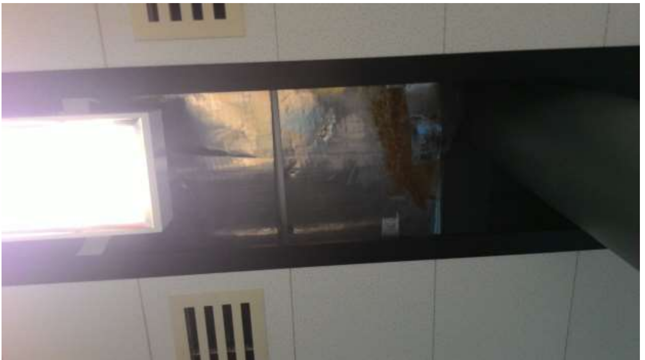
Diagram 26: Discoloration of fibrous insulation
