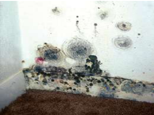
Figure 11: Mould growth in a closet due to condensation of room air (Owners, 2006)
