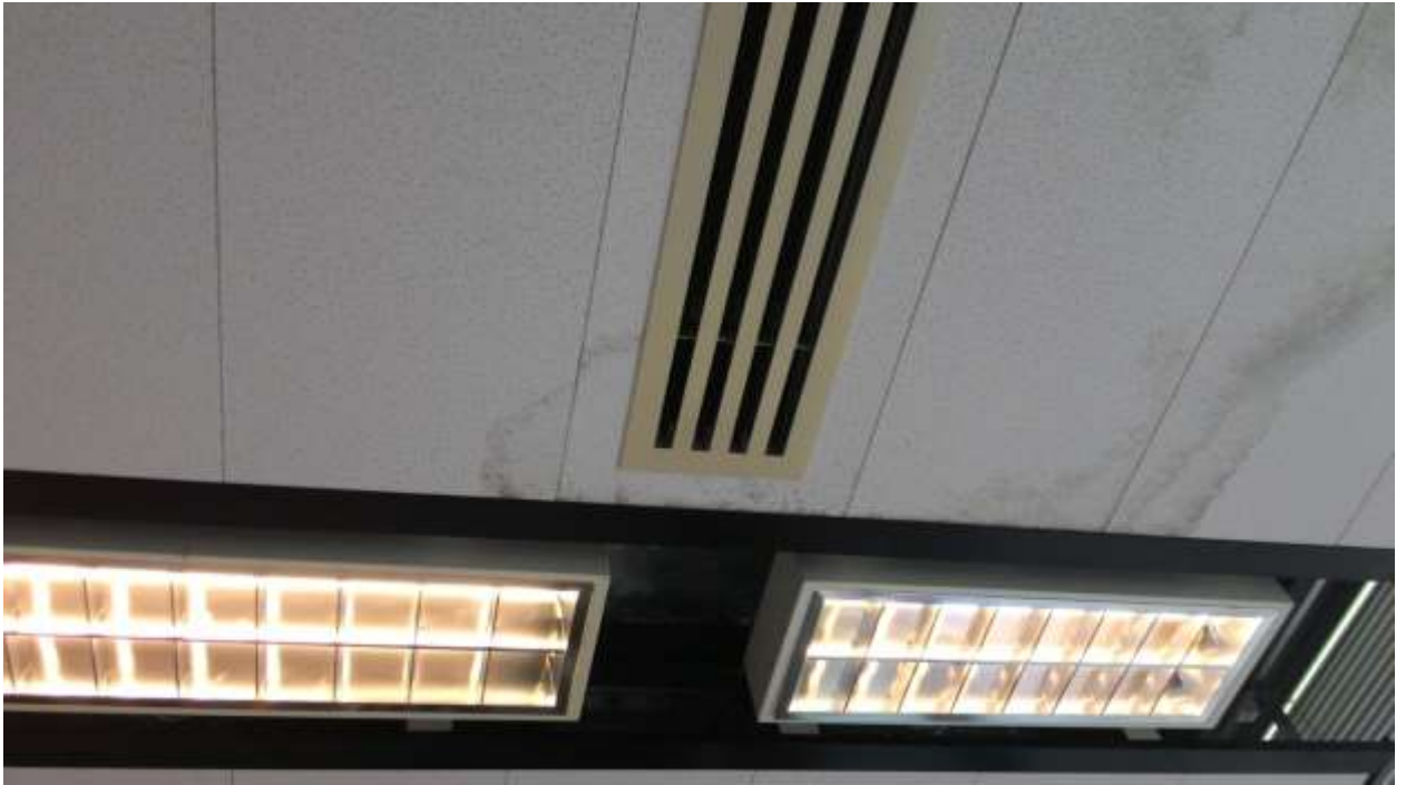
Diagram 7: Water seepage marks found at the ceiling
