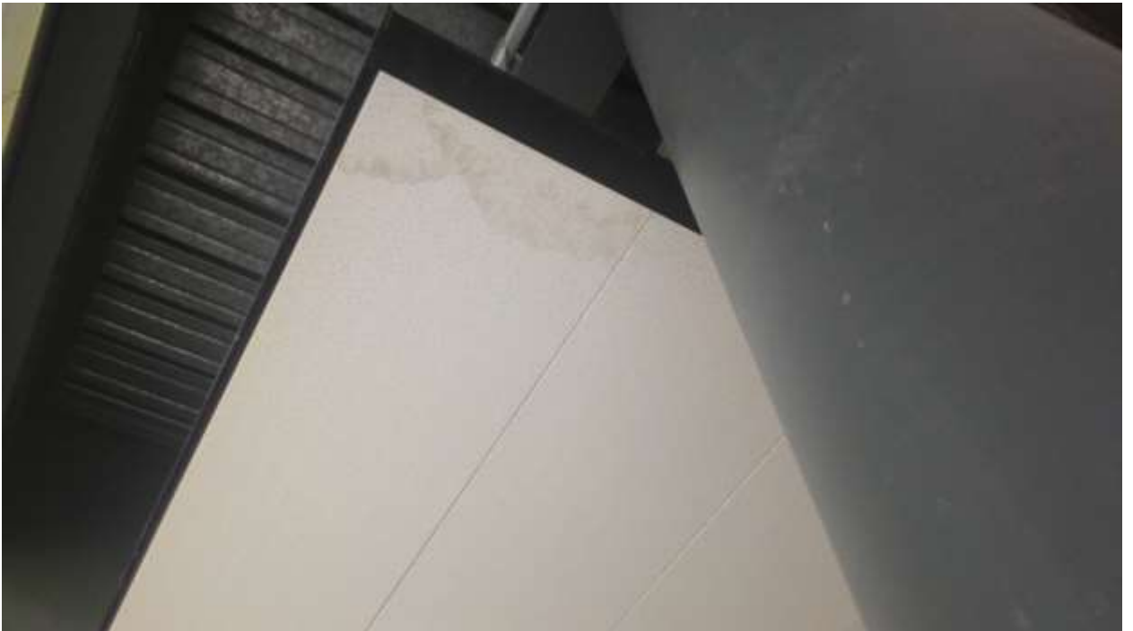
Diagram 12: Water seepage marks found at the ceiling
