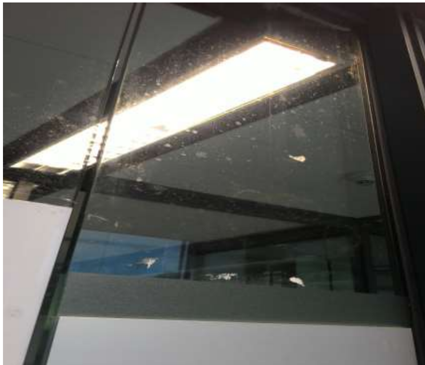
Diagram 34: Mould stains found on the glass door panel
