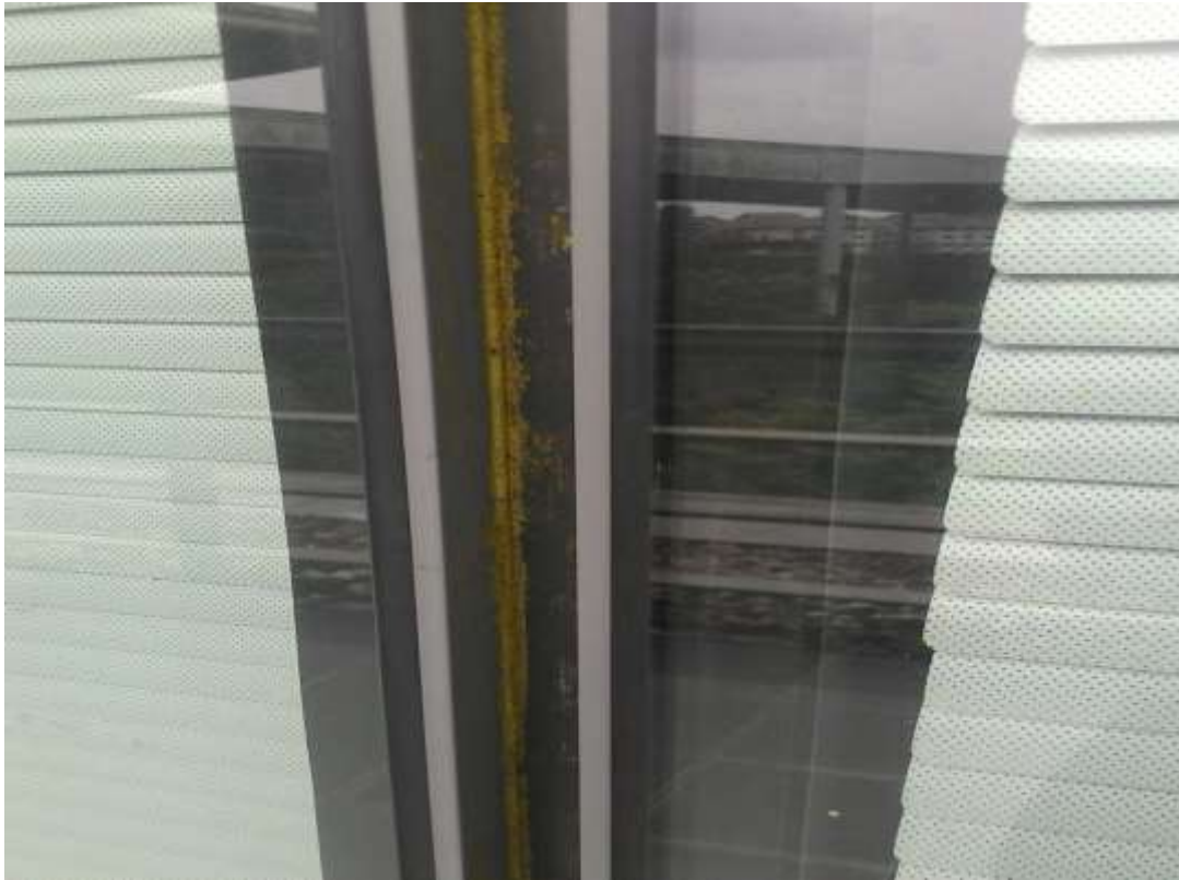
Diagram 29: Mould contamination at the edge of windows ( building exterior )
