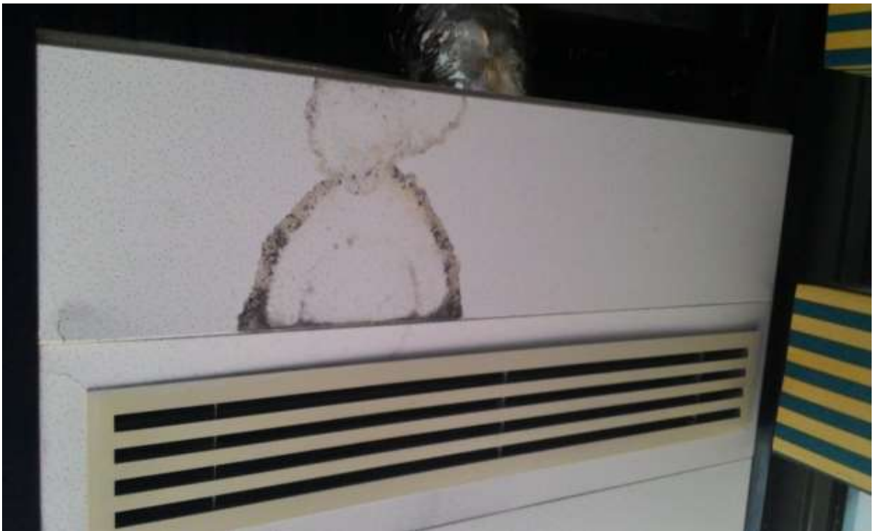
Diagram 14: Mould contamination spotted due to excessive water seepage
