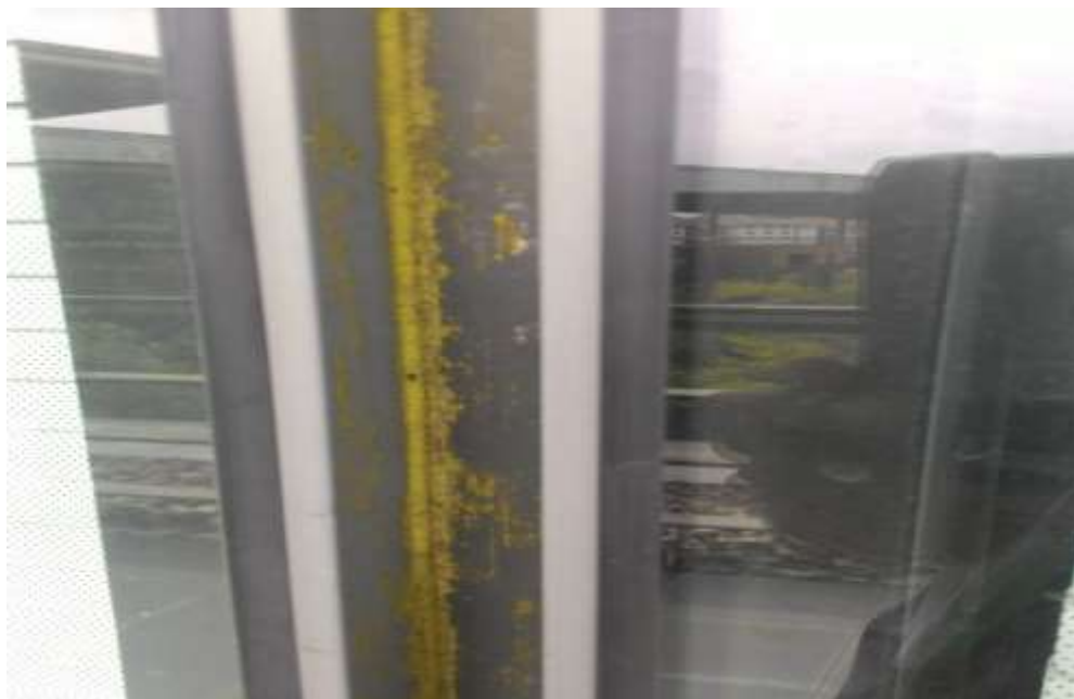
Diagram 30: Mould contamination at the edge of windows ( building exterior )
