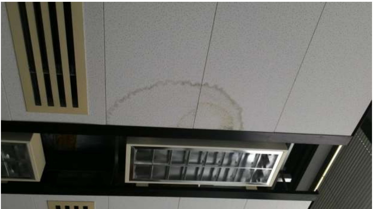
Diagram 8: Water seepage marks found at the ceiling
