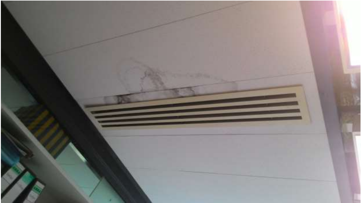
Diagram 13: Mould contamination spotted due to excessive water seepage
