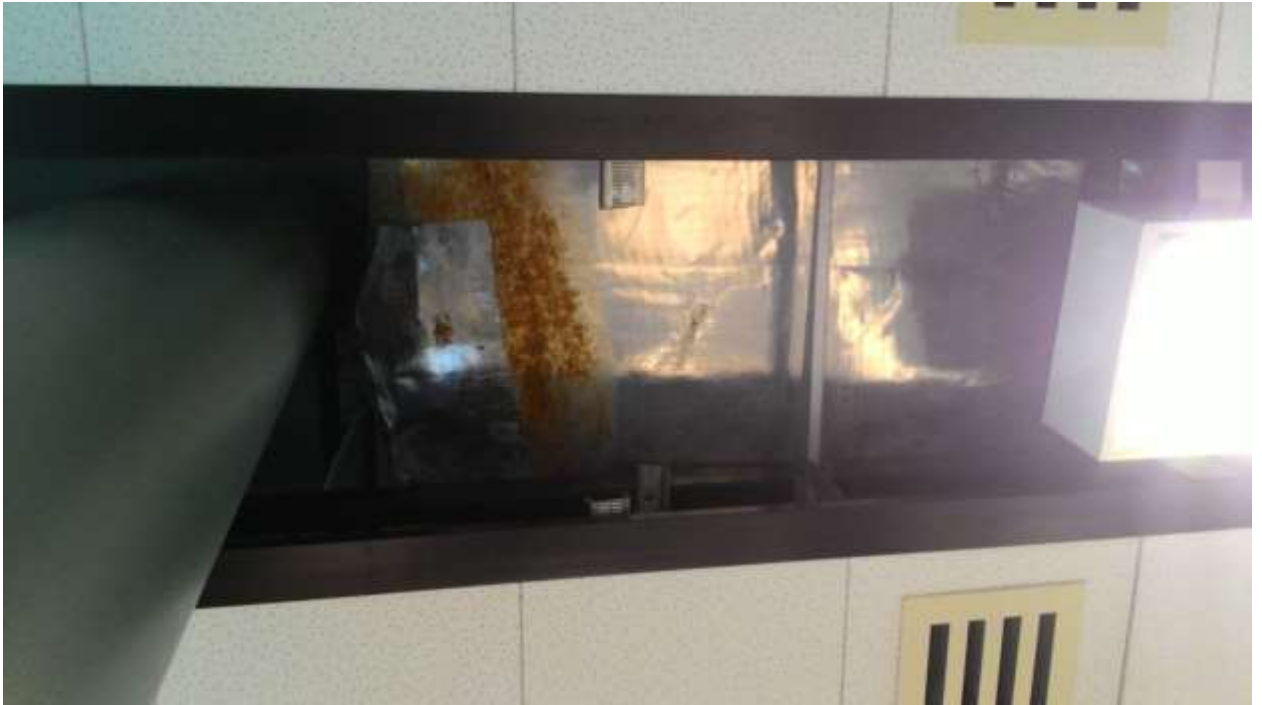
Diagram 27: Discoloration of fibrous insulation
