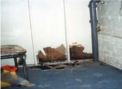
Figure 13: Mould growth at the back side of wallboard (Owners, 2006)
