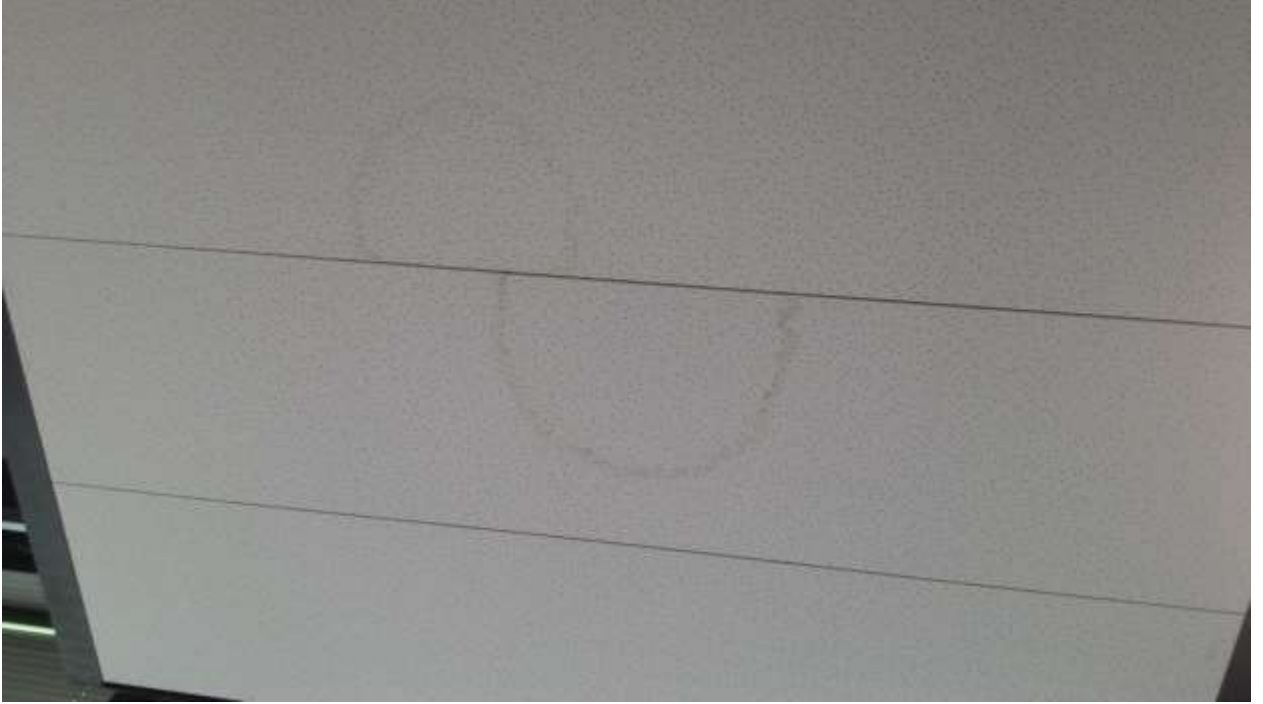
Diagram 11: Water seepage marks found at the ceiling
