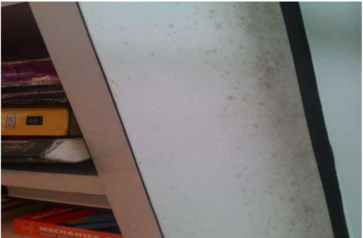
Diagram 18: Mould found at the exterior of cupboards
