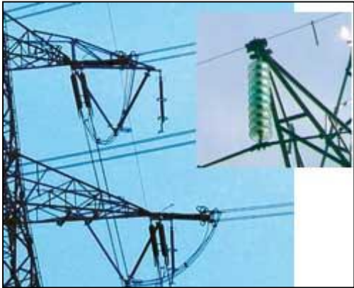
Figure 8. Lightning Surge Arrester on Transmission Line
