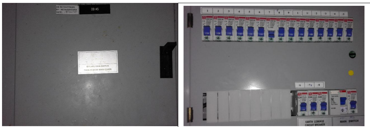
Figure 5: V4-D T1 Panel Box
