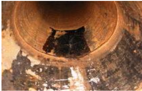
Figure 1.1: Internally corroded oil pipeline [1]
