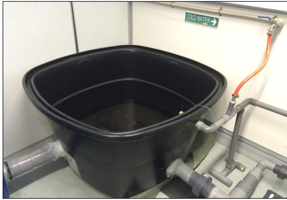
Appendix 2.1: The supply water tank and the water inlet source.
