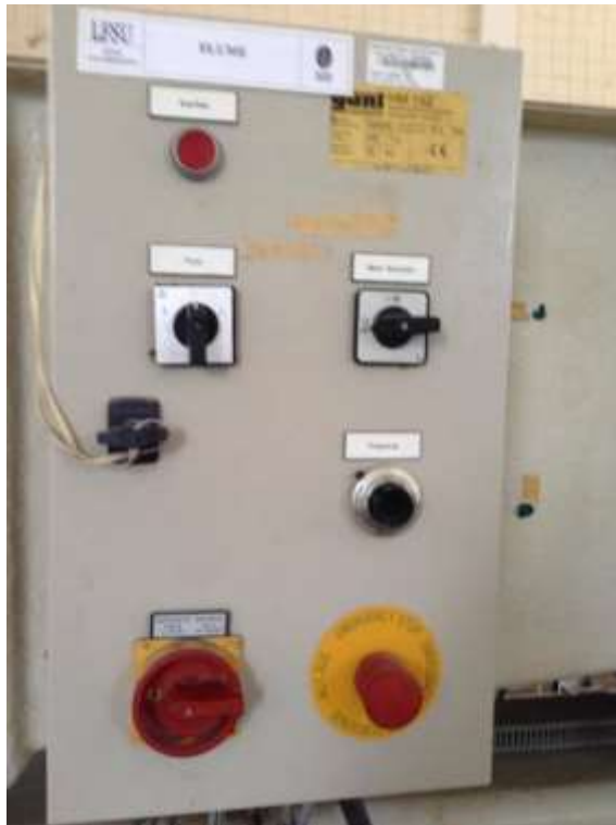
Figure 3.7: Controllers for frequency, wave generation and pump.
