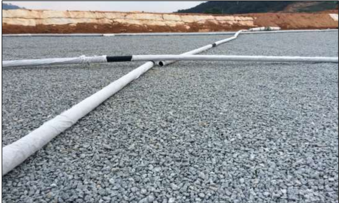
Figure 3.1: Network of Subsoil Pipe Installed during the Final Cover Layering
