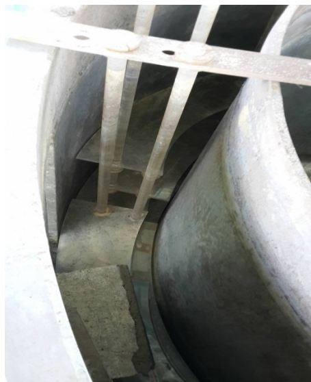
Figure 13: Installed baffle in clarifier unit
