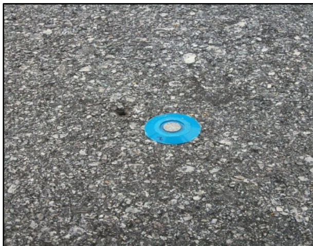
Figure 3.3: Surveying Nail and Survey Marker Disc
