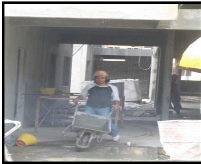
The worker did not wear proper PPE
