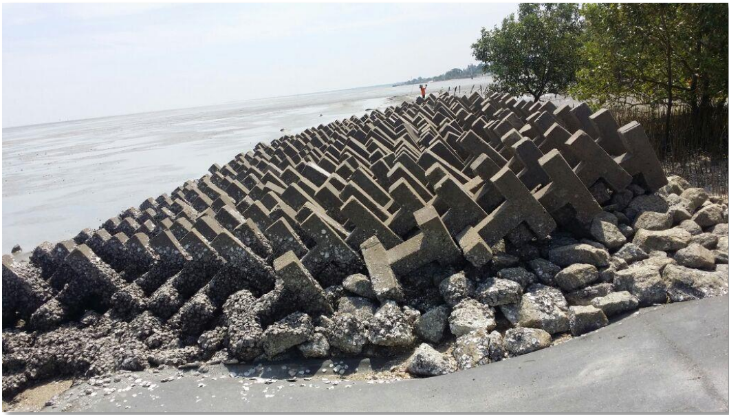
Figure 3.2: SAUH revetment was constructed on top of the Geotube breakwater
