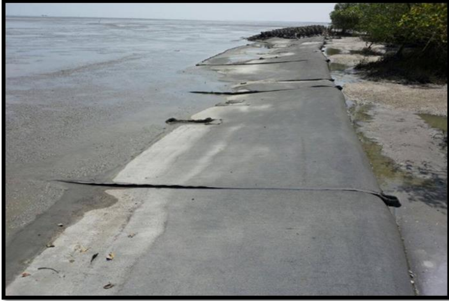
Figure 2.3: Example of geotube condition in Sungai Haji Dorani now in 2016
