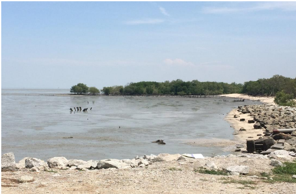
Figure e: The current site condition at Sg. Haji Dorani, Selangor
