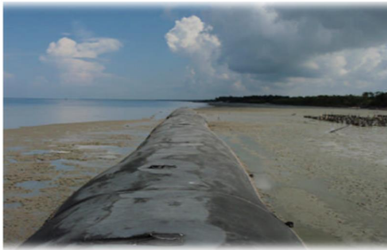
Figure 2.2: Example of geotube used in Sungai Haji Dorani, Selangor, Malaysia
