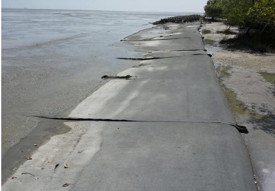
Figure f: The current condition of geotube breakwater at Sg. Haji Dorani, Selangor
