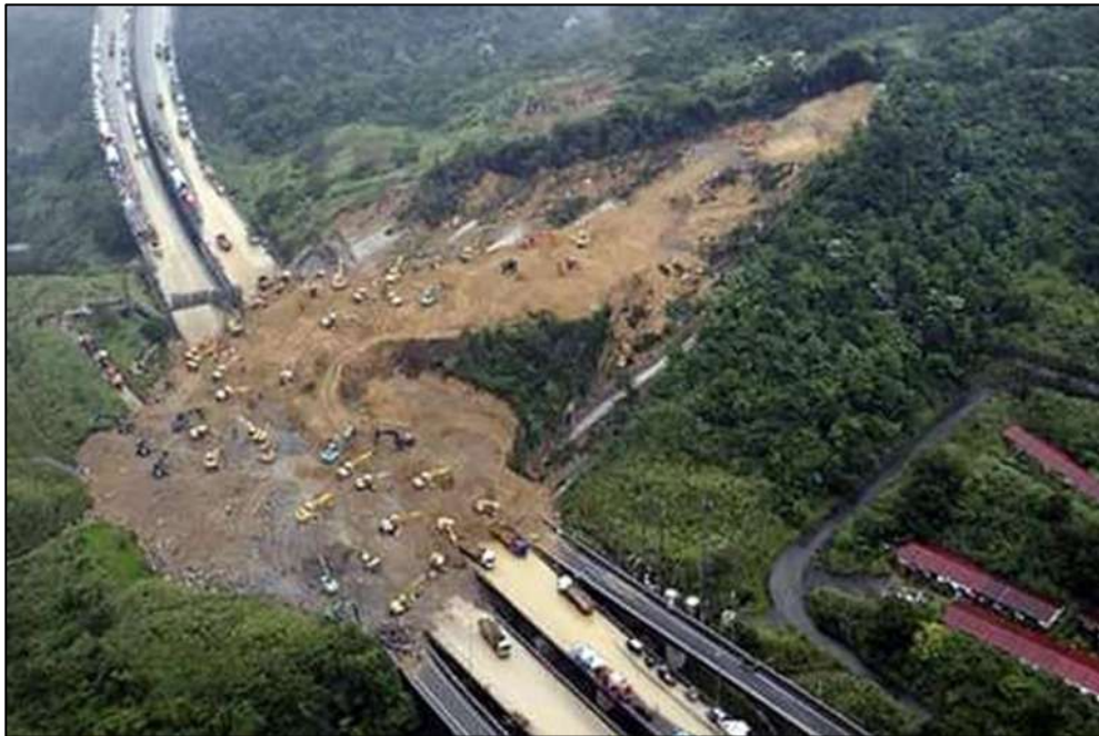
Figure 2.1: Karak Highway Landslide on Nov 11, 2015 (source: google image)
