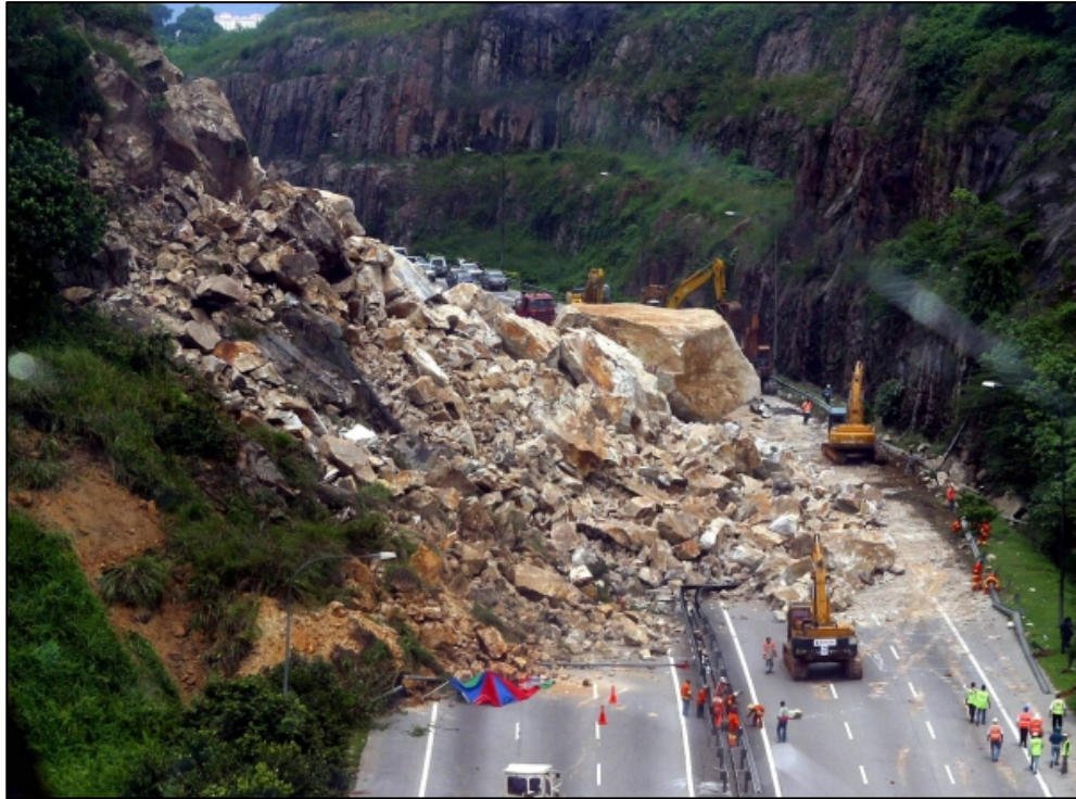
Figure 2.2: Bukit Lanjan Landslide (source: google image)
