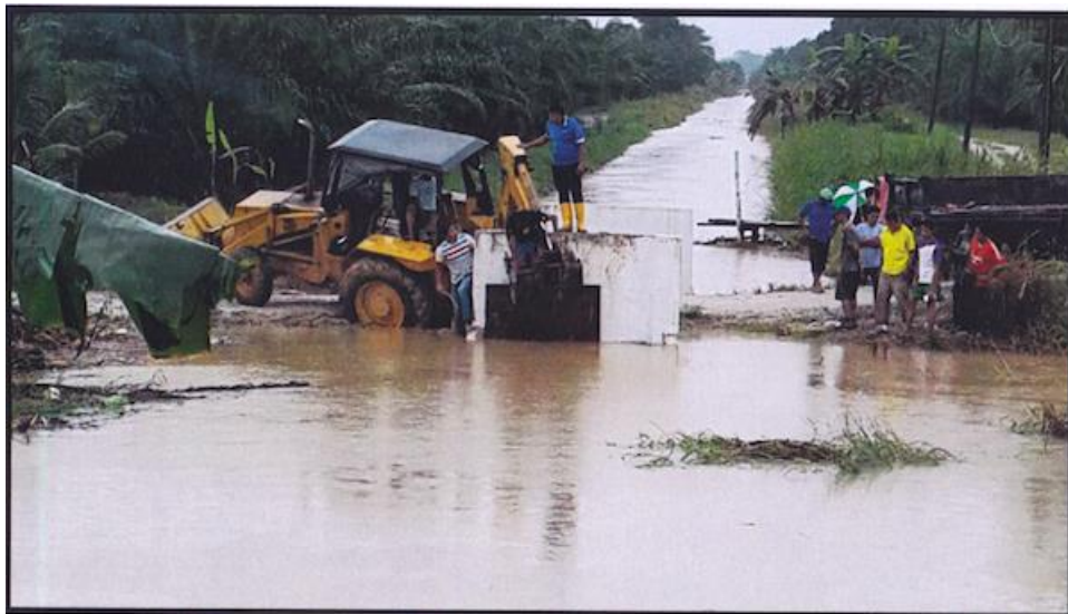
Figure 22: Works of Reinstalling Water Gates (Source: JPS Ipoh)
