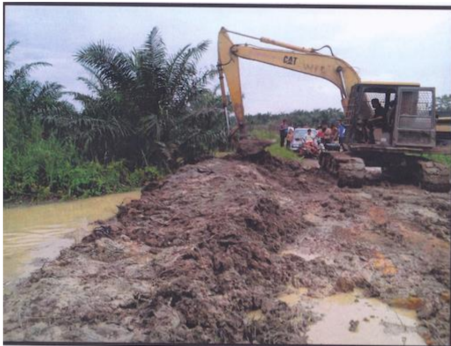
Figure 24: Topping Up Bunds Along Perak River
