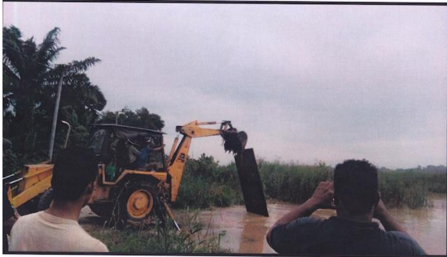
Figure 23: Installation of Chequered Plates
