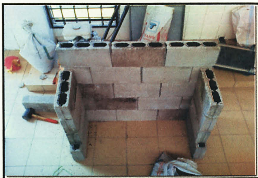
Figure 3.20: Completed prototype crumb rubber noise barrier wall with crumb rubber filler and side wall
