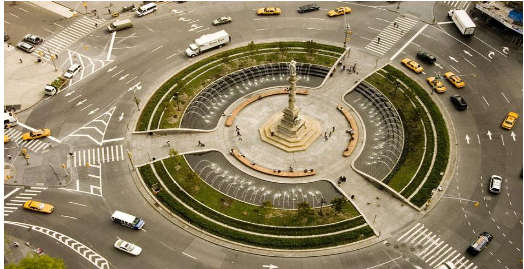
FIGURE 6: Roundabout (NYC: Department of Design and Construction, 2014)
