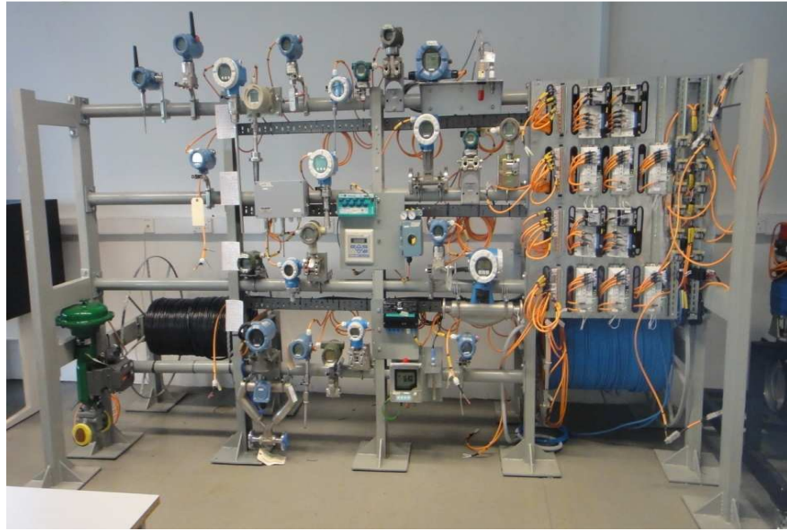
Figure 13: Foundation Fieldbus devices after upgrading
