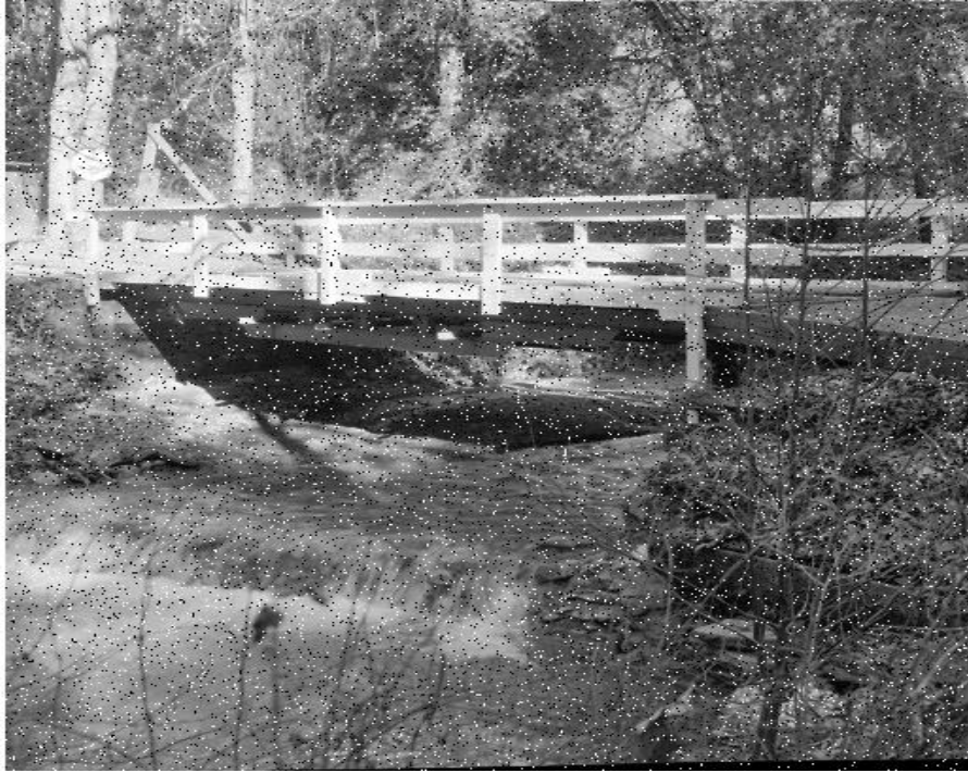
Figure 52: Bridge corrupted with Salt and Pepper noise at variance 0.05
