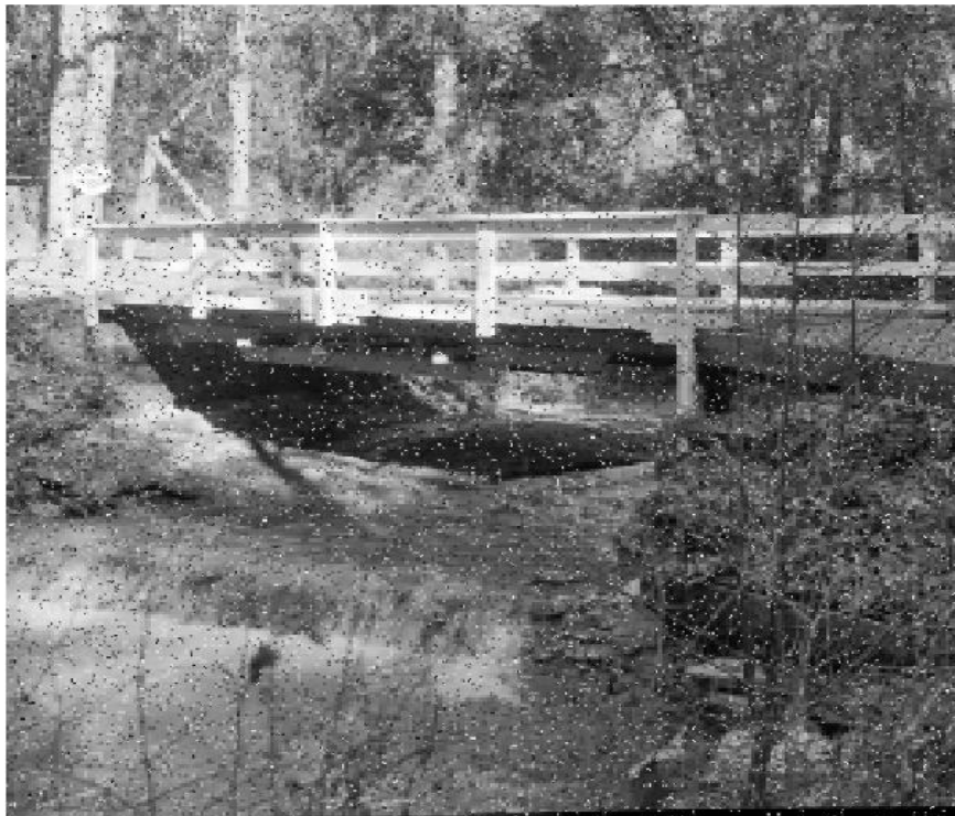
Figure 53: Denoised Bridge using Haar at level 3
