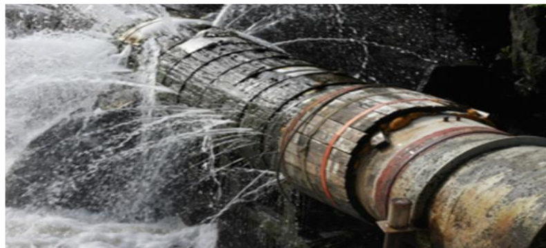
FIGURE 1.1: Piping System Leakage
