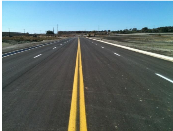
Figure 2: Asphaltic Concrete Highway.
