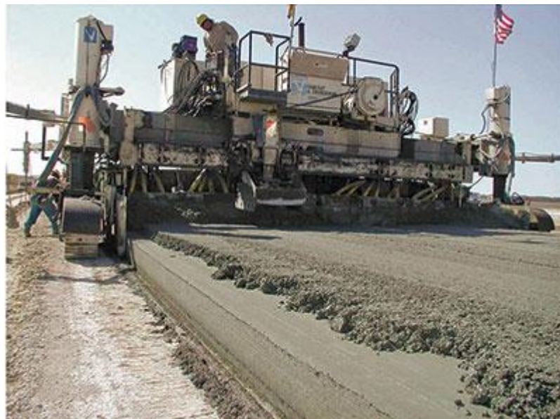
Figure 6: Geopolymer Concrete Paver Machine.
