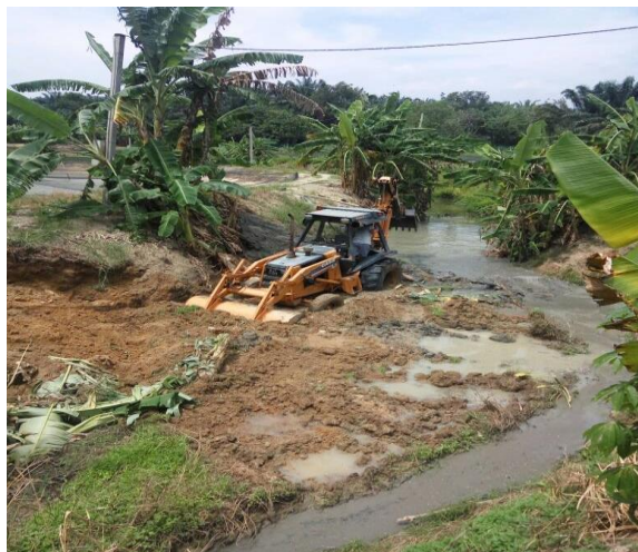
Figure 5: Channel Excavation Works
