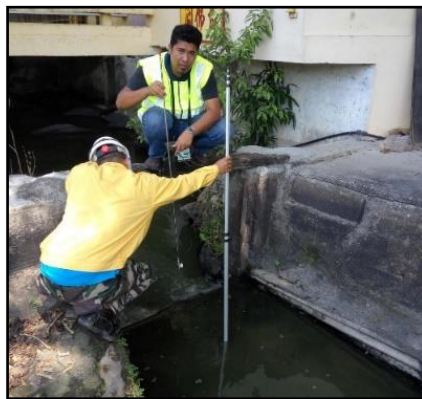
Figure 17: River Profiling Work
