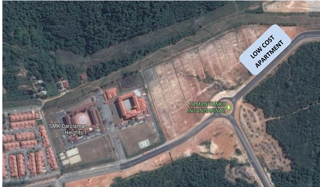
Figure 1.5.2: Taman Tunku Intan Safinaz (Fasa-1) Low Cost Apartment in Jitra, Kedah,
