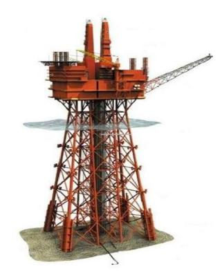
FIGURE 2 TYPICAL FIXED PLATFORM (ICF INCORPORATED, 2015)
