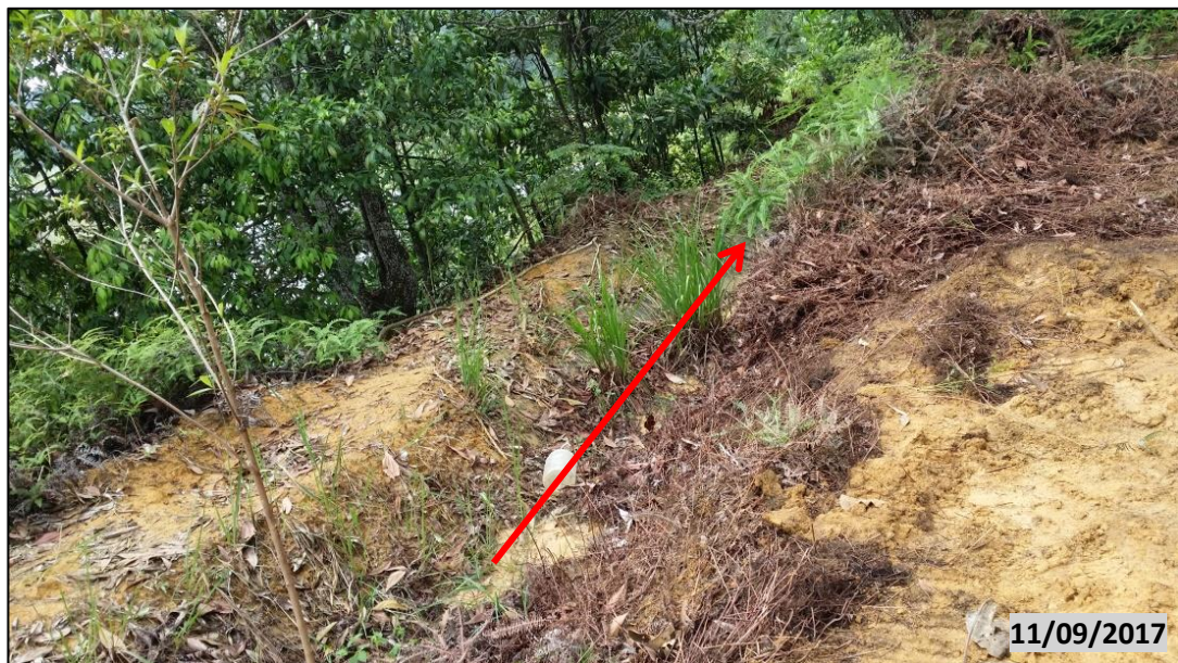
Figure 4-1: Clogged Drain ( Source: Author )
