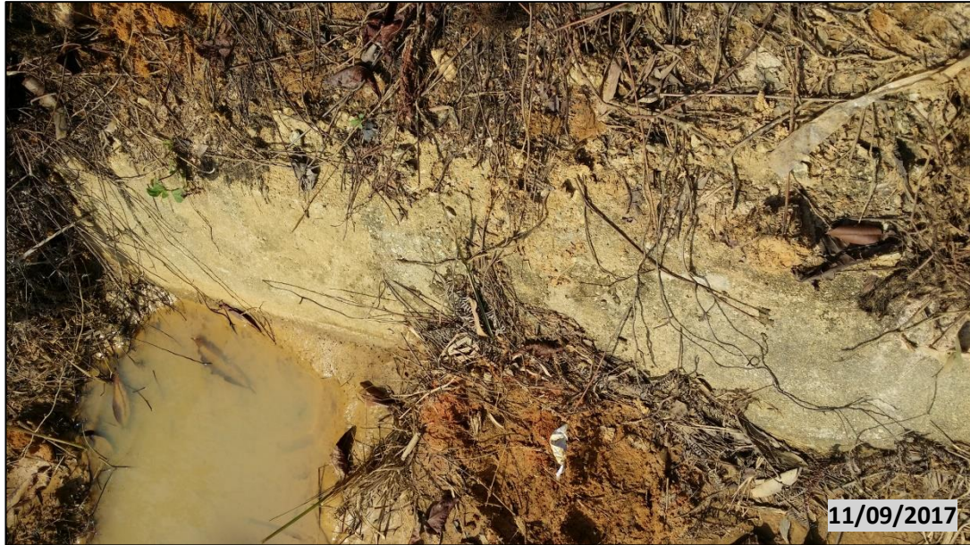
Figure 4-2: Stagnant Water in the Drain (Source: Author)
