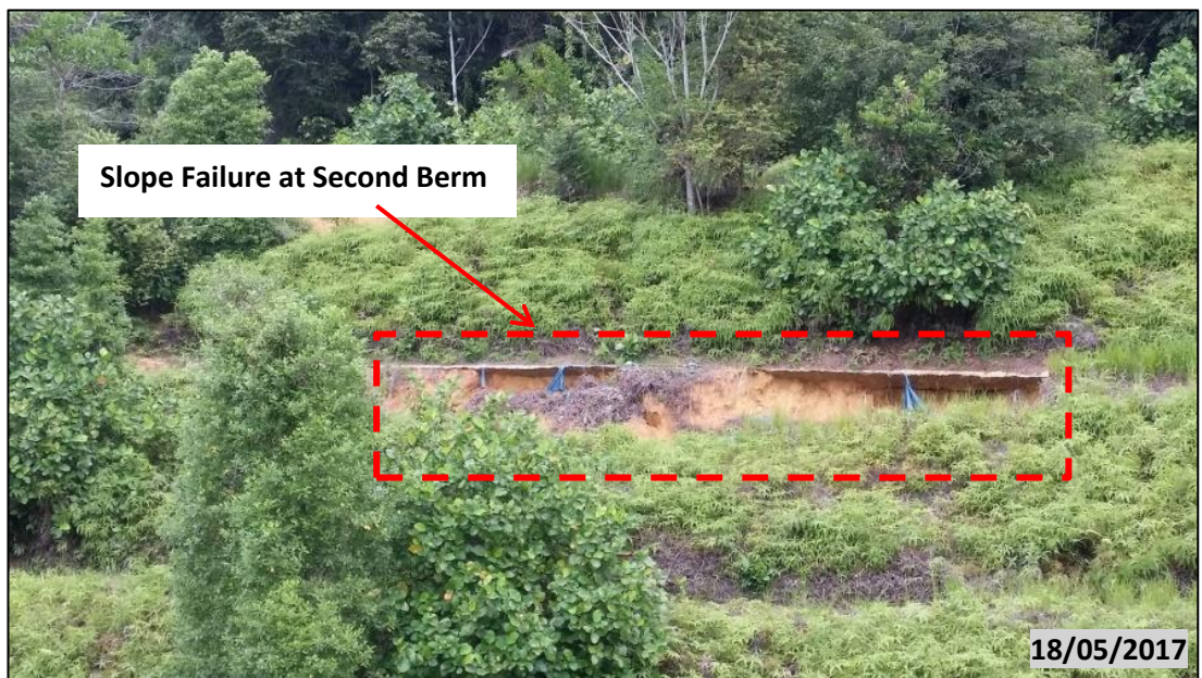
Figure 1-2: Slope Failure View from Block 14 (Source: Author)
