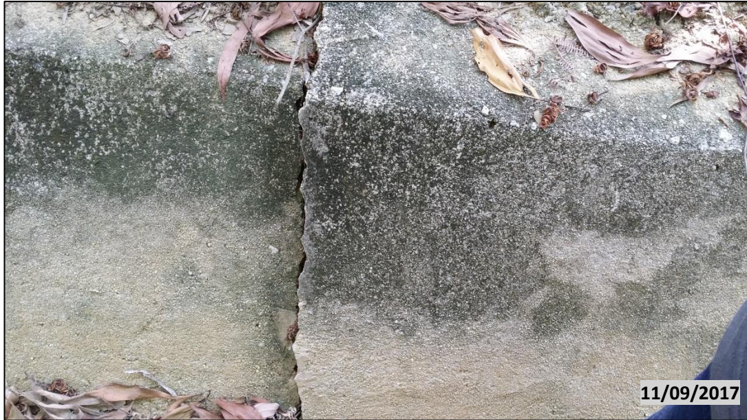
Figure 4-4: Cracked Drain ( Source: Author )
