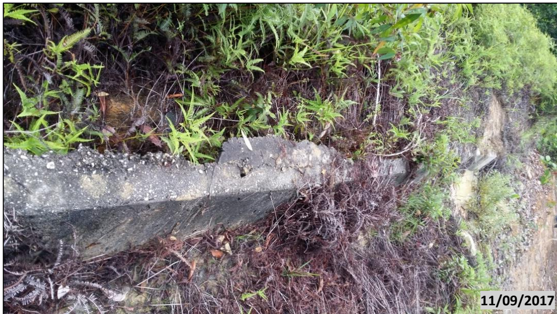
Figure 4-3: Misaligned Drainage (Source: Author)
