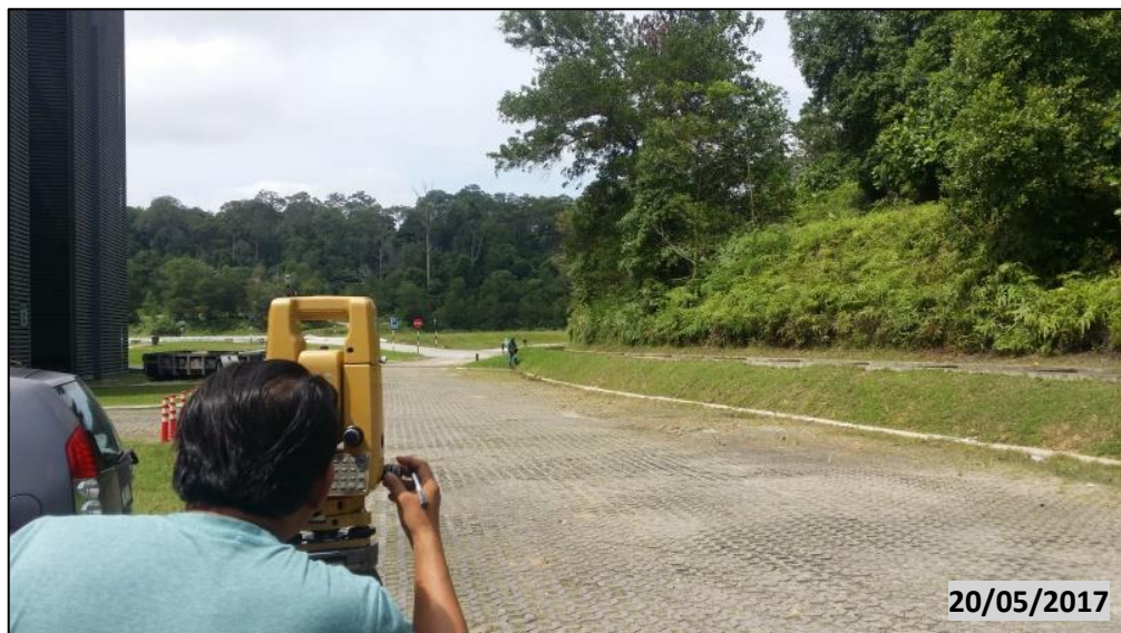
Figure 3-2: Collecting the Coordinates using a Total Station (Source: Author)
