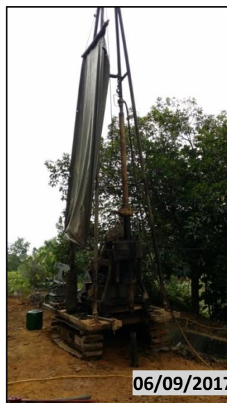
Figure 3-6: Rotary Wash Boring (Toho D2K) (Source: Author)
