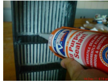
Figure 3.15: Sealing the joint with silicon sealant
