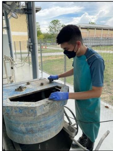
FIGURE 3.2: Mixing of 35 MPa Ordinary Concrete
