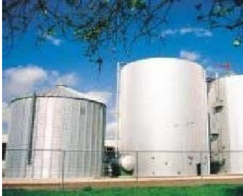
Figure2: The sewage sludge digesters at Tilburg Plant in the Netherlands
