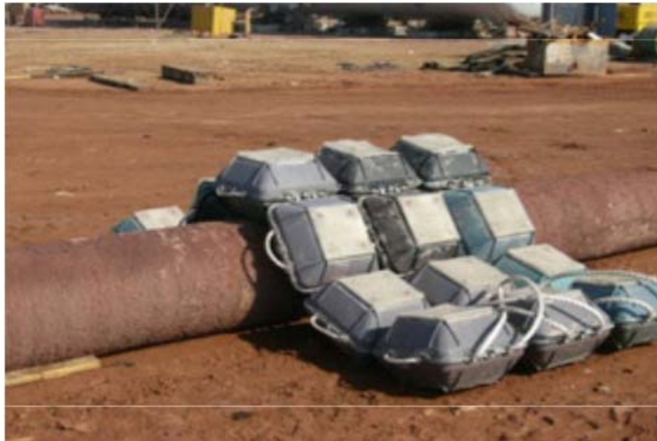
Figure 2: Secondary stabilization – concrete mattresses [13]
