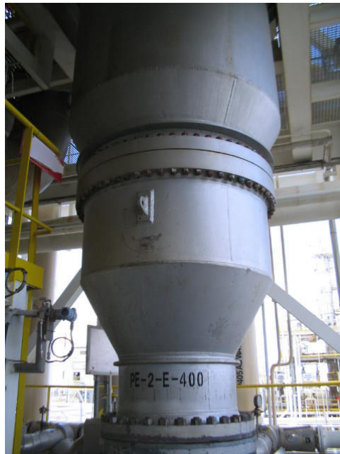
Figure 2.10: PE-2-E-400 Heat Exchanger in EPMSB
