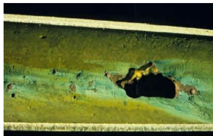
Figure 2.6: Inner surface having Erosion Corrosion
