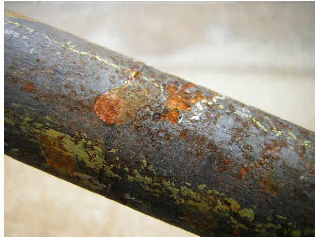
Figure 2.12: Tube sheet having deep pitting
