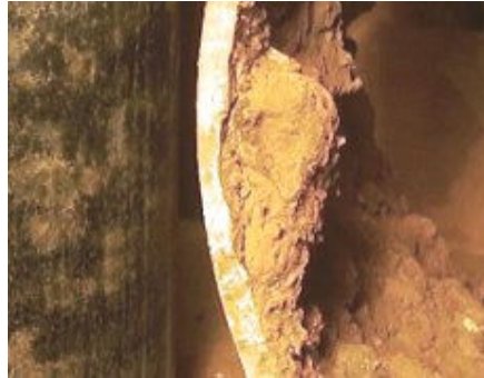
Figure 2.7: Deposit at inner surface of tube
