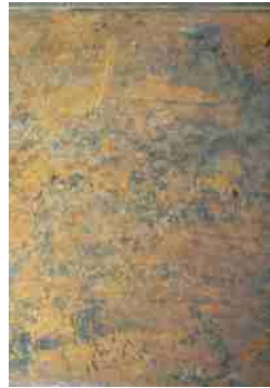
Figure 2.2: Showing corrosion at tube surface
