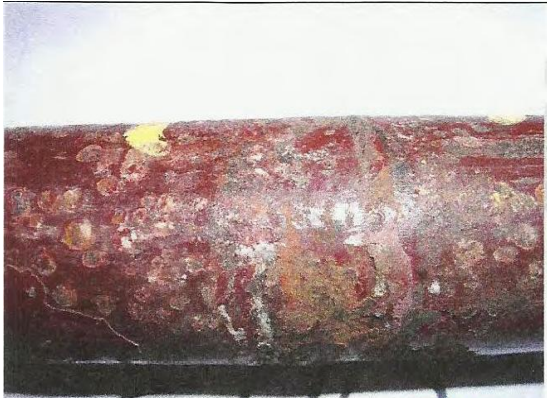
Figure 4.1: As received E-105 with coating damage/blister on tubing external [6]
