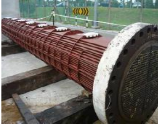
Figure 4.14: Touched-up peeled off coating after the contractor did hydro-jetting due to some damaged peeled off the existing coating [12]
