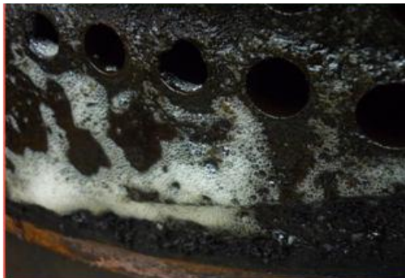
Figure 4.18: Sticky blackish deposited noted entire tube sheet surface [12]
