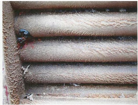
Figure 3.2: Thick brownish/slimy deposit/fouling observed next to tubing and baffle plate intersection [6]
