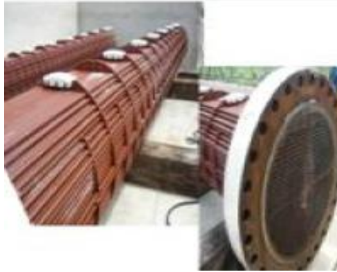
Figure 4.12: View of tube bundle noted in satisfactory condition. No sign of any abnormalities observed [12]
