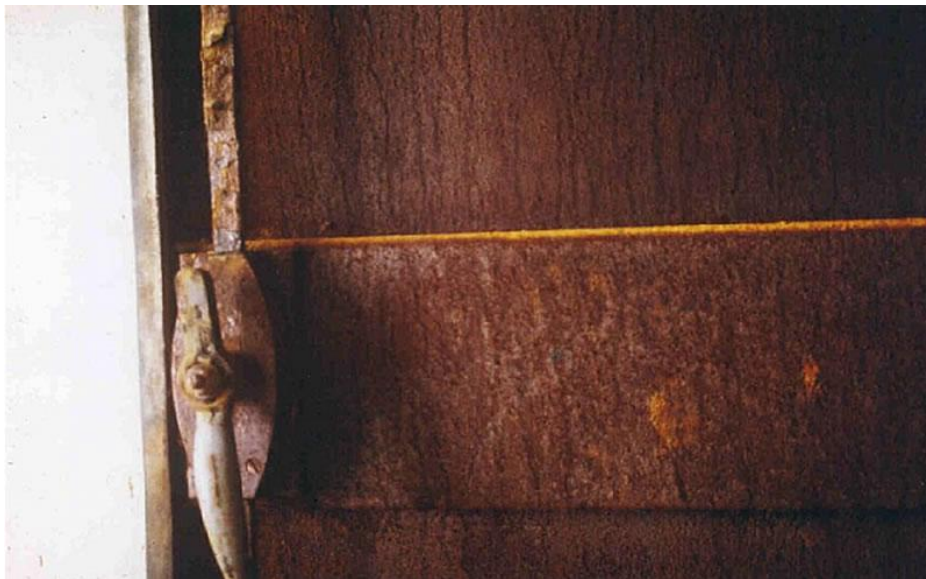
Fig. 2.5 Corrosion of a ferritic stainless steel door in a sulphur-containing atmosphere
