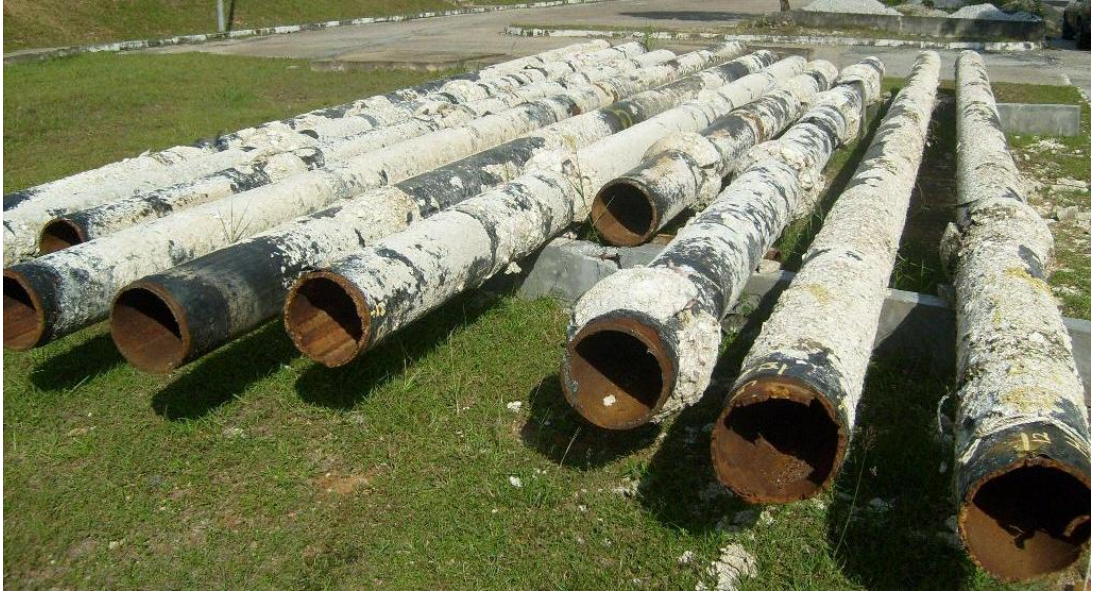
Plate D.1 Sections of abandoned pipeline
