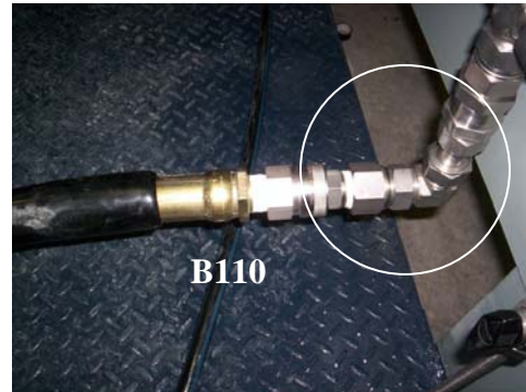
(b) The other end of flexible hose is coupled to inlet of regulator.
