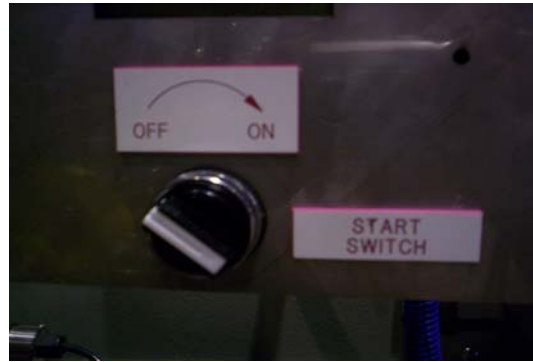
(b) Switch located on display panel is turned to 'ON' position.
