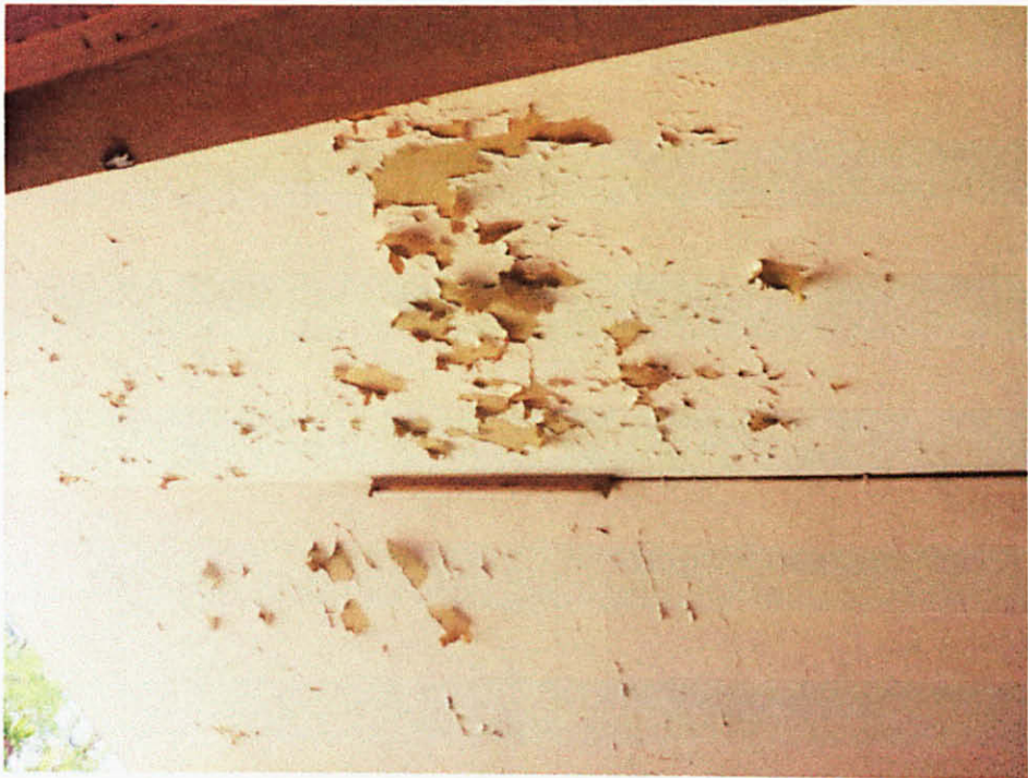
Figure 2: Peeled off ceiling paint
